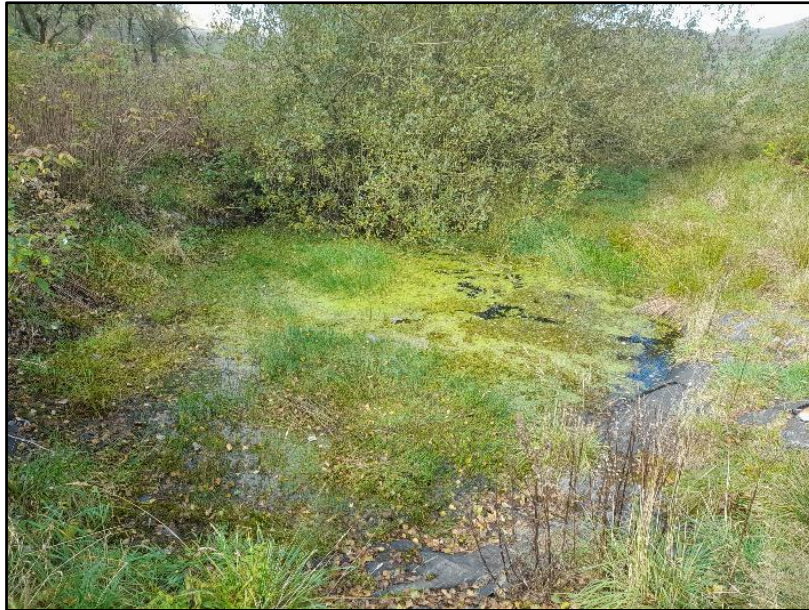
Figure 29. Pond, with low water level and exposed liner.
