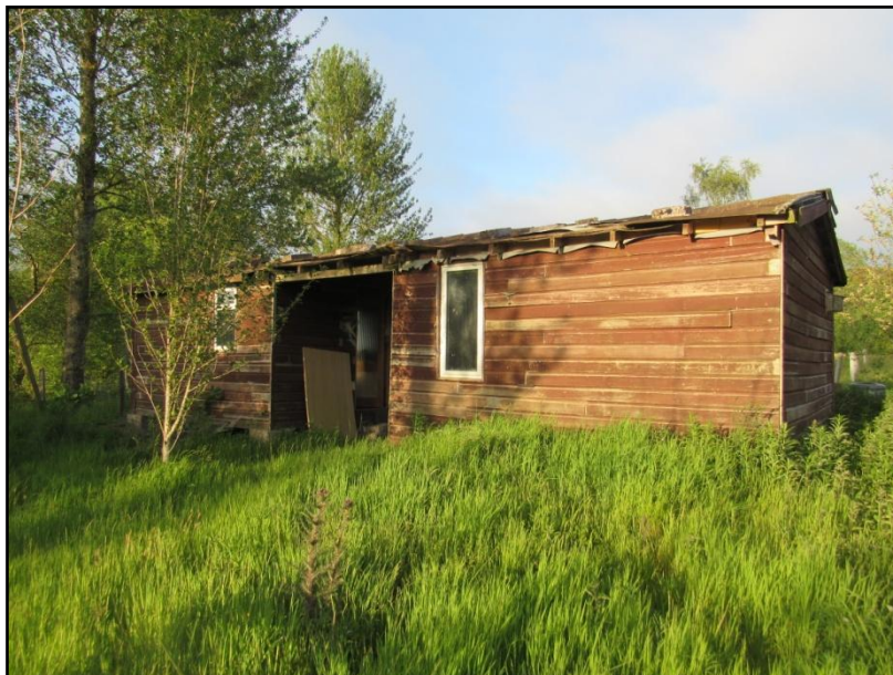
Figure 18. The Shed – western elevation.
