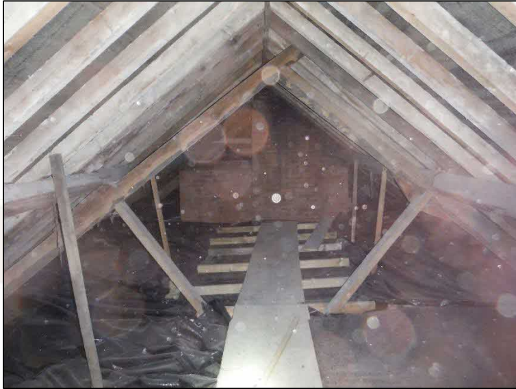
Image 1: Retained and enhanced (6no access tiles, maintenance/monitoring walkway) brown long-eared bat loft in Building 1.
