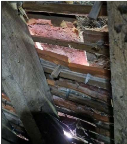
Image 19. Internal view of exposed clay tiles found throughout the north-south facing roof void.
