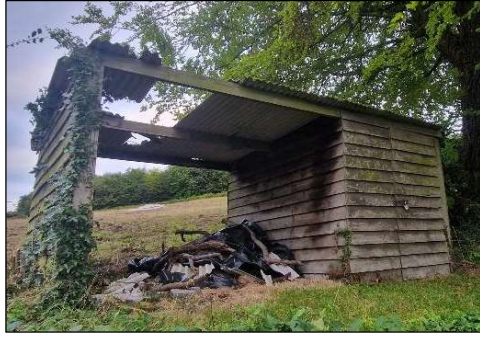
Image 22. View wooden outbuilding from the front.
