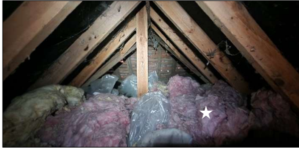
Image 17. View of main void heading west from the hatch access.
