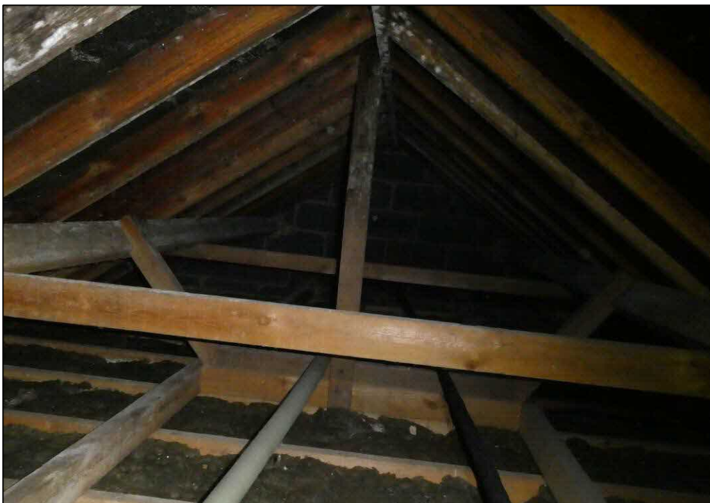
Figure 16. Internal space of Loft 2. Southernwood, Woolton Hill. 21.03.23
