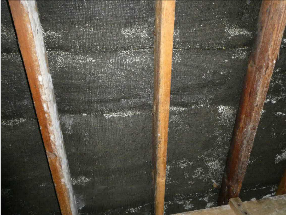
Figure 13. Example of bitumen lining in Loft 1. Southernwood, Woolton Hill. 21.03.23
