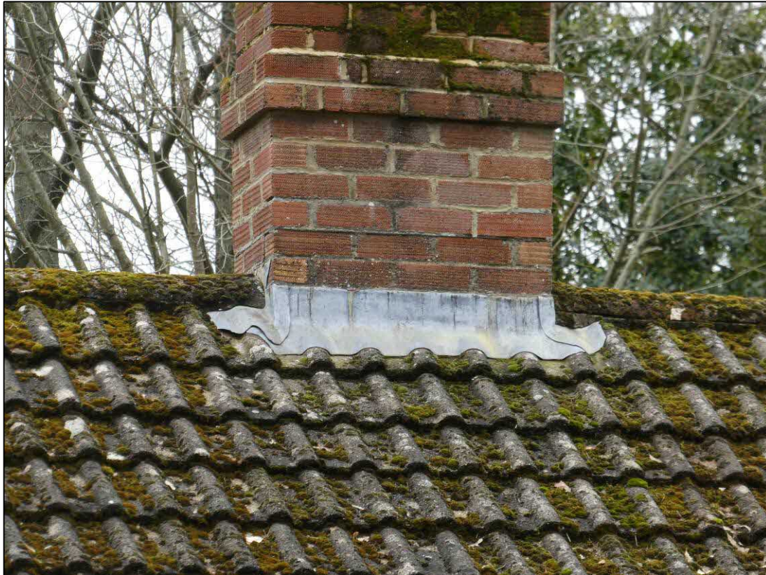
Figure 6. Tightly fitted lead flashing. Southernwood, Woolton Hill. 21.03.23
