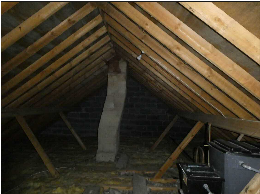
Figure 12. Internal space of Loft 1. Southernwood, Woolton Hill. 21.03.23
