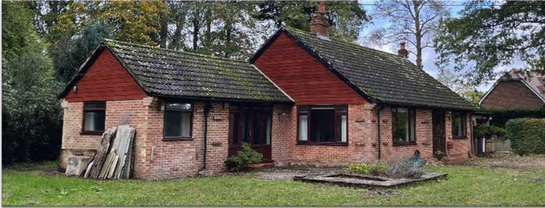
House to be demolished.
