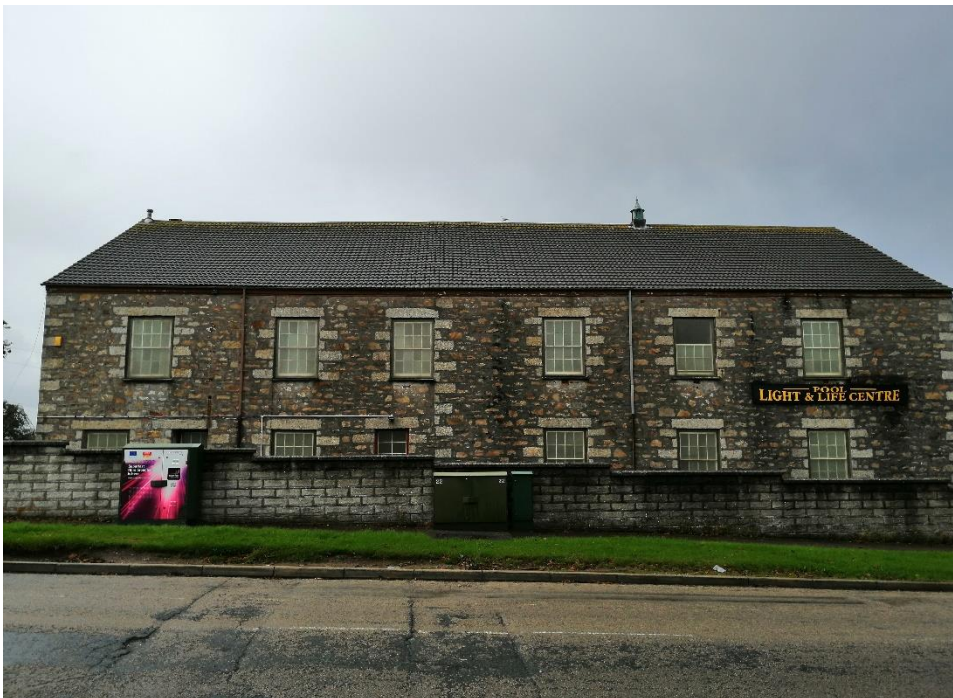
East elevation as viewed from Wilson Way
