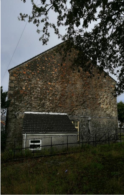
South elevation. Showing the single storey modern kitchen extension
