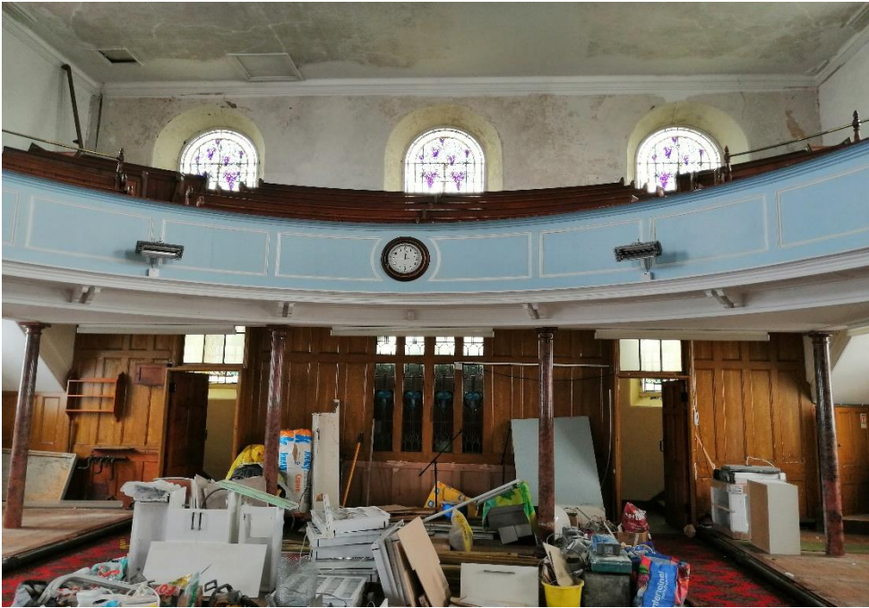
Looking North showing entrance screen with gallery over.
