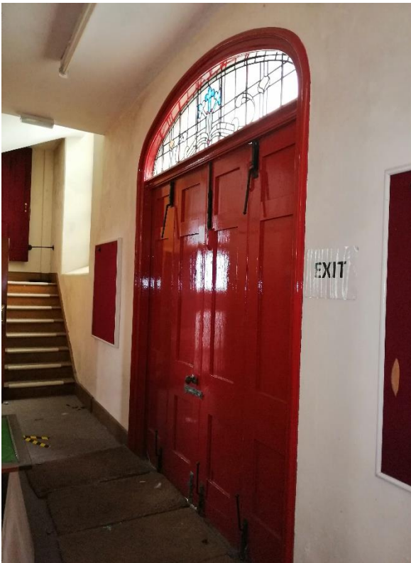
Showing main entrance door & overlight to North elevation
