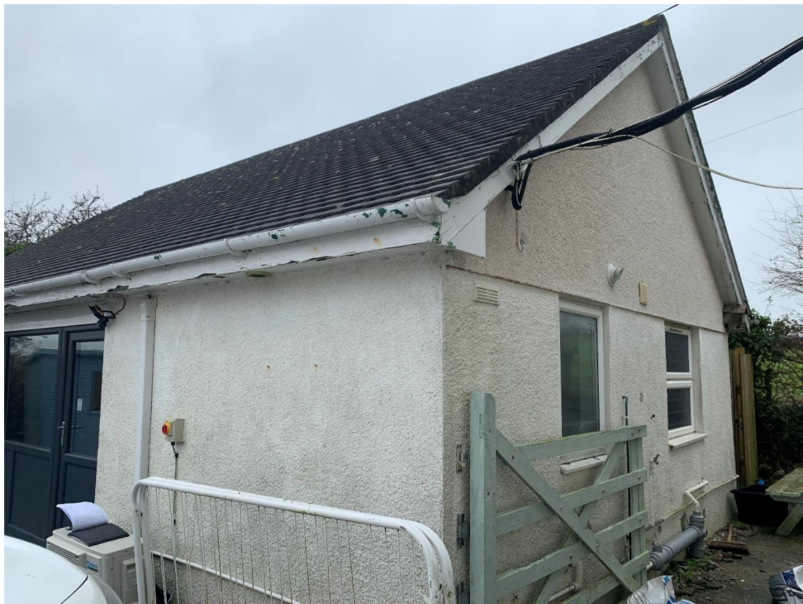
Figure 1: Southern elevation of building assessed
