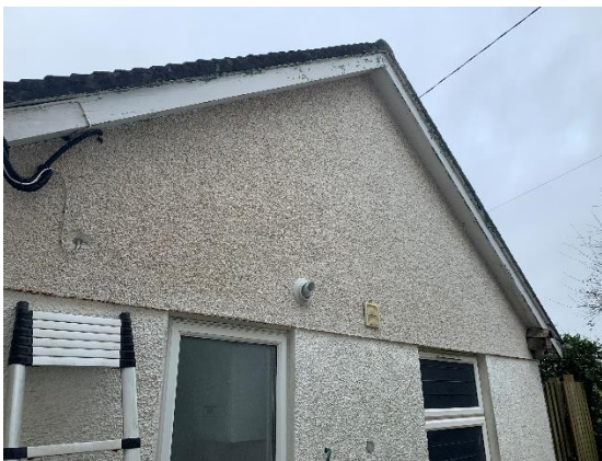
Figure 2: Eastern gable end of annex
