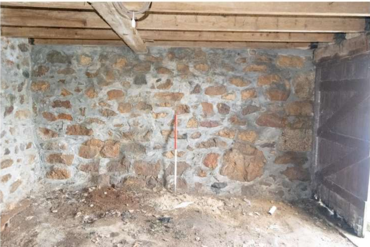
iii) Looking northwest
