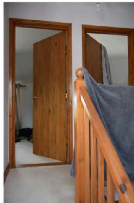
v) First floor modern stud walls and doors Archive ref:CHENH0821_0048.JPG
