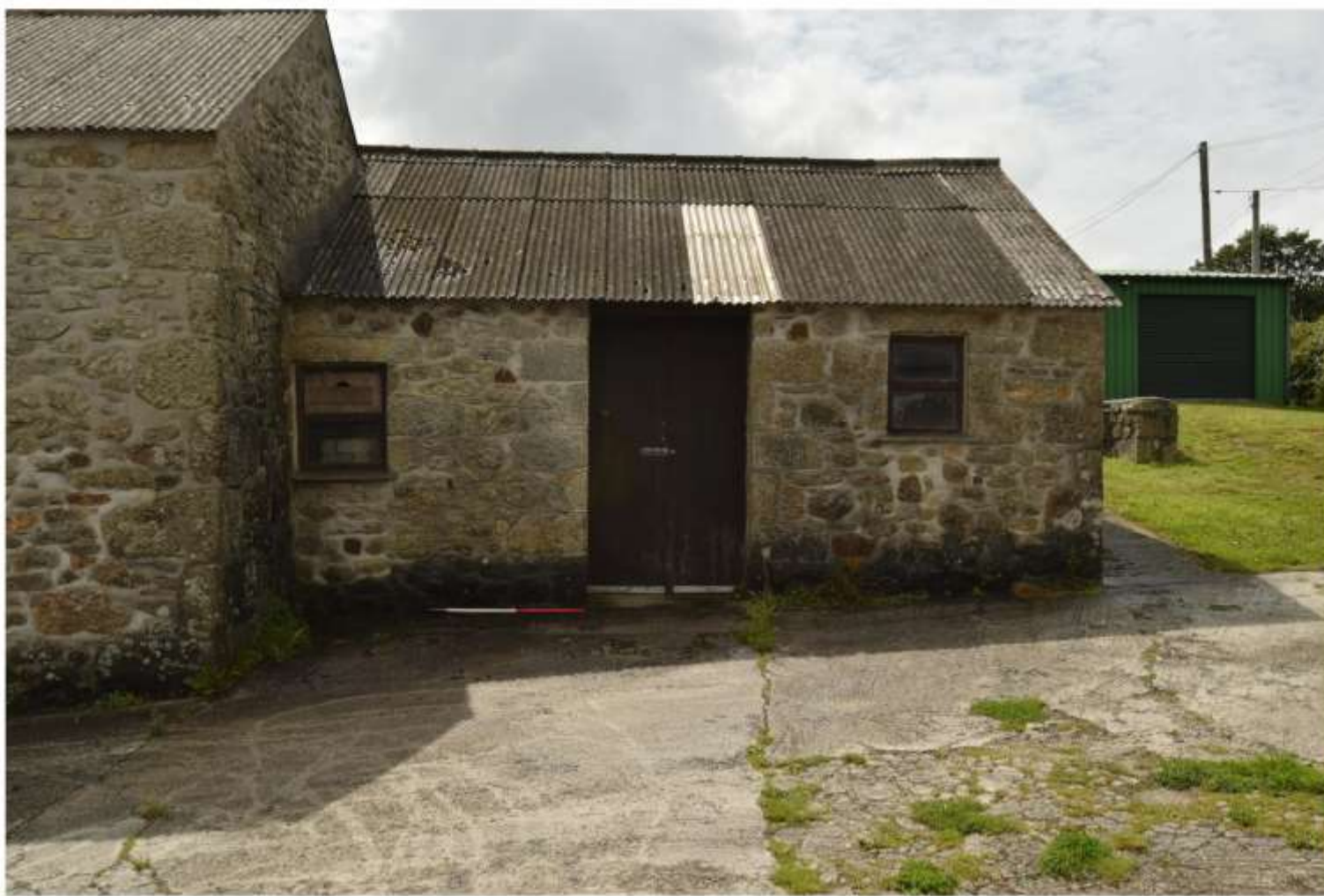
i) Northeast elevation Archive ref: CHENH0821_0365.JPG Scale 1m
