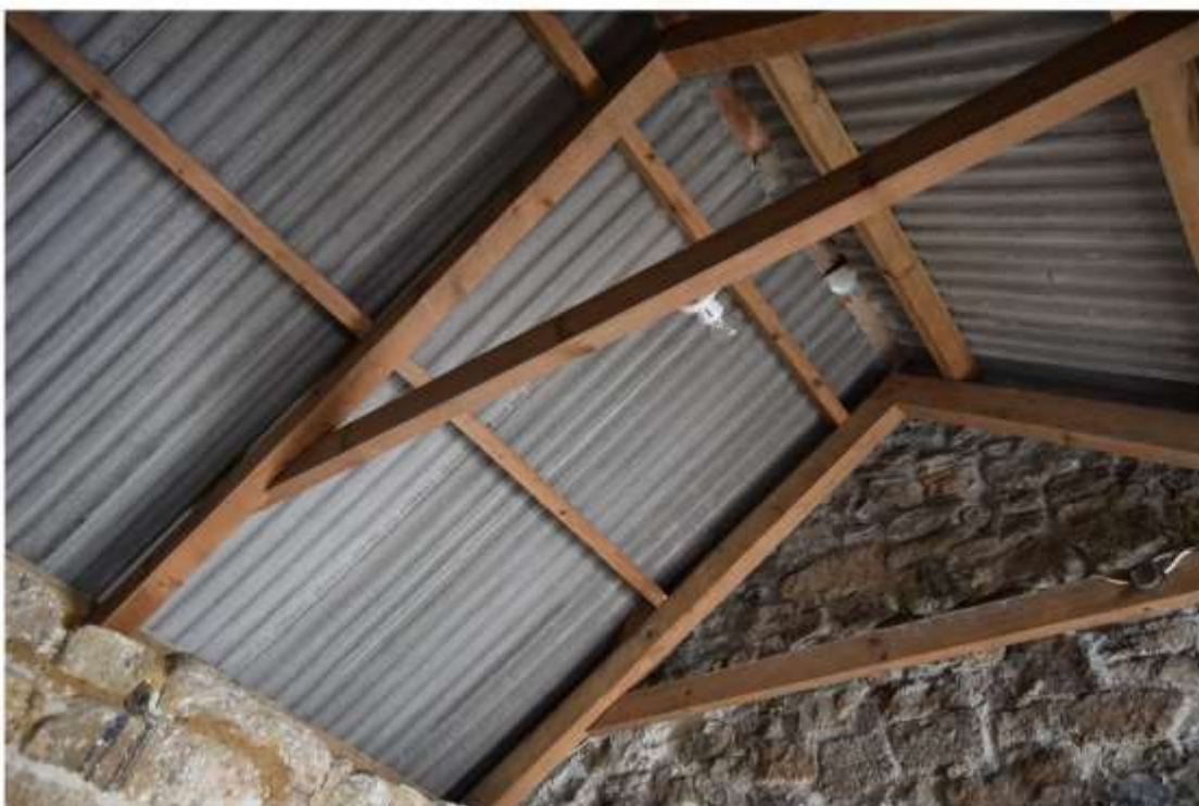
iv) Looking west, roof structure Archive ref: CHENH1223_0073.JPG
