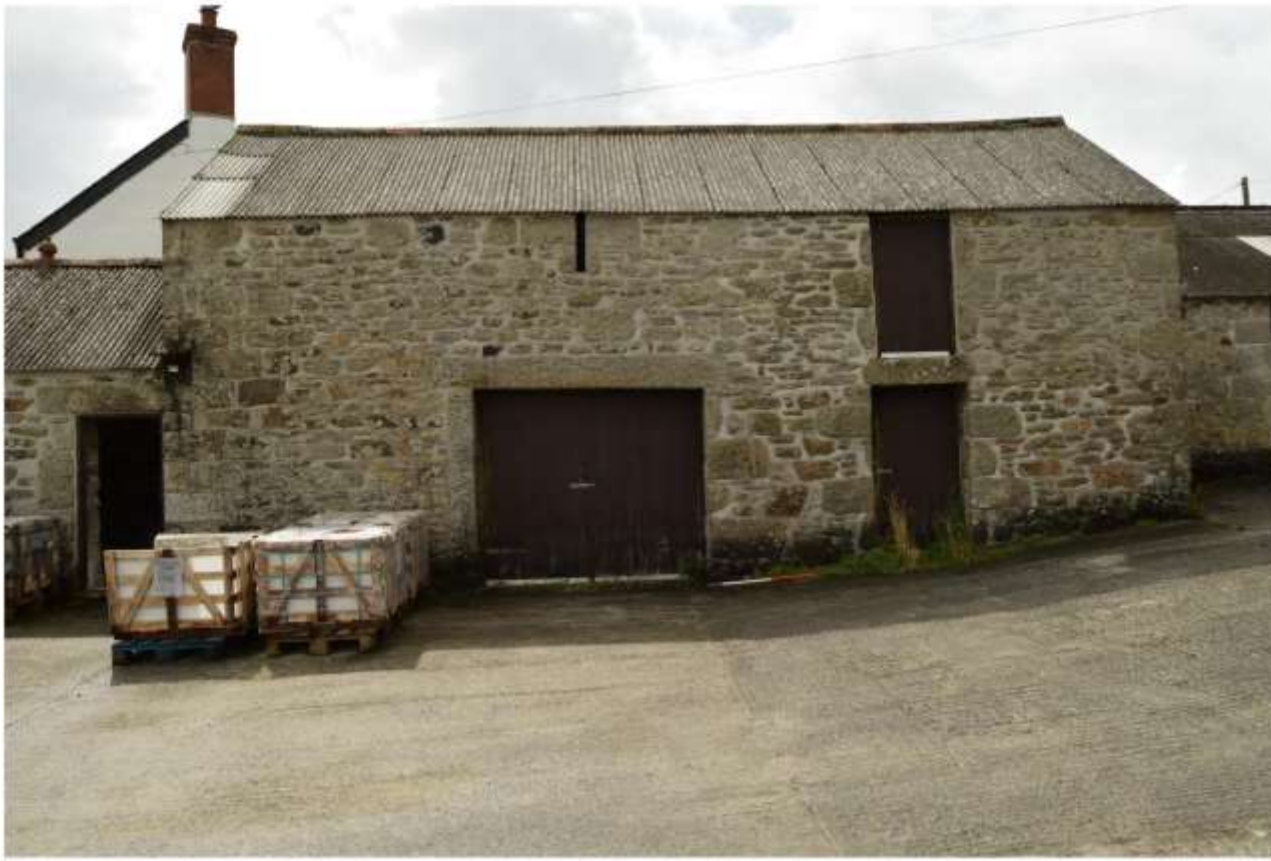
i) North east elevation Archive Ref: CHENH0821_0364.JPG Scale 1m
