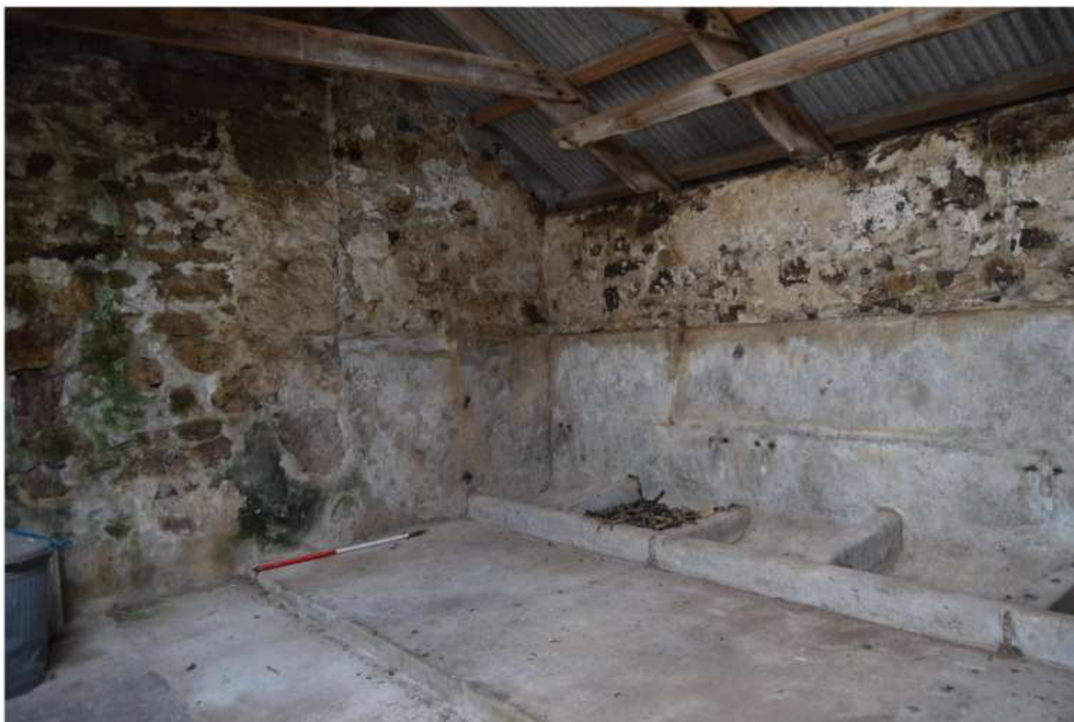
iii) southwest wall and roof structure Archive ref: CHENH0821_0026.JPG Scale 1m
