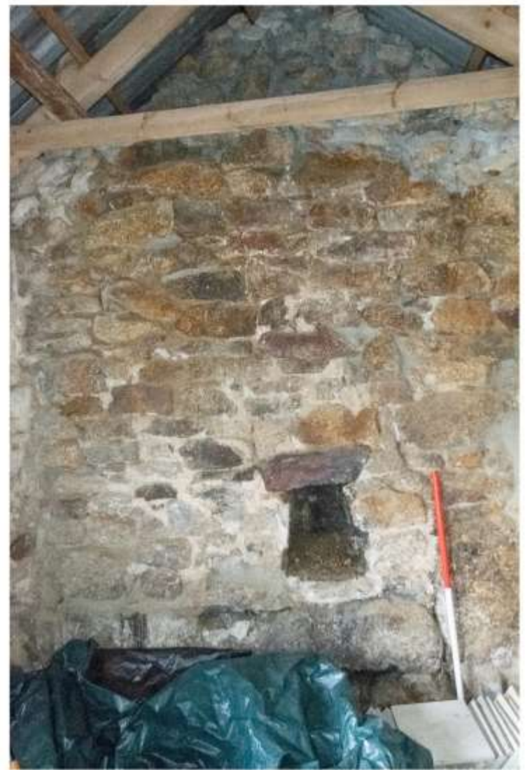
ii) Southeast wall, showing lantern niche Archive ref: CHEN1223_0070.jpg Scale 1m
