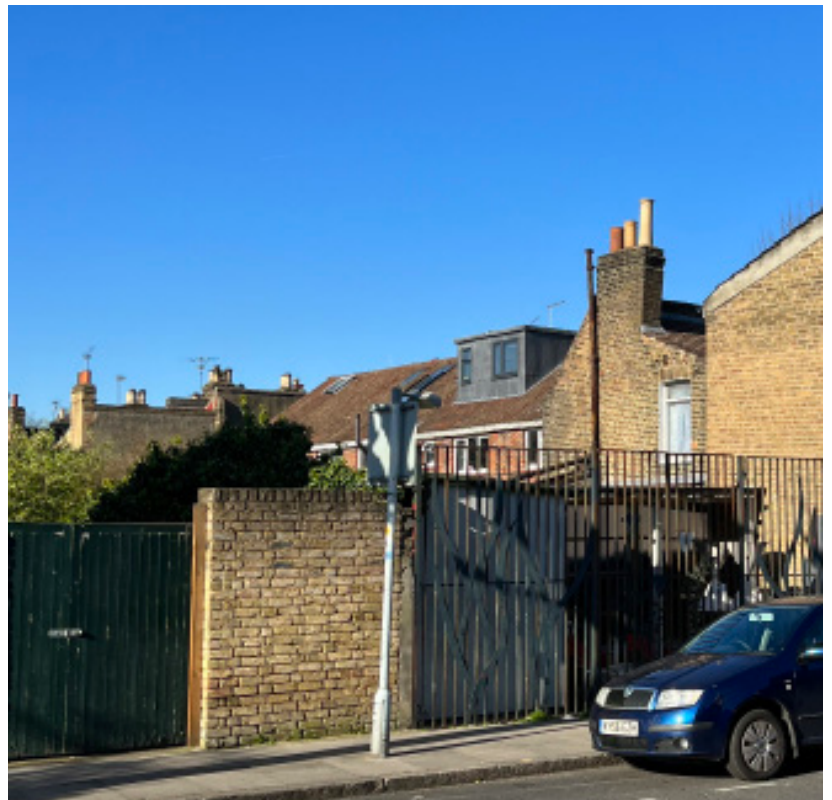
At 134 Bellenden Road a dormer roof extension has been constructed despite this property being in the same heritage area
