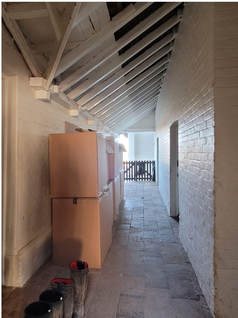
Fig. 5. Corridor between the main house and the workshop wing.
