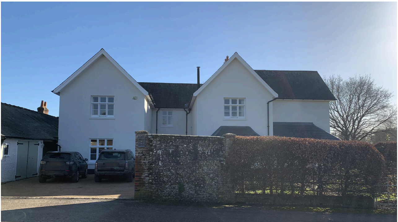
Fig. 2. Lane side notional 'front' of main house.
