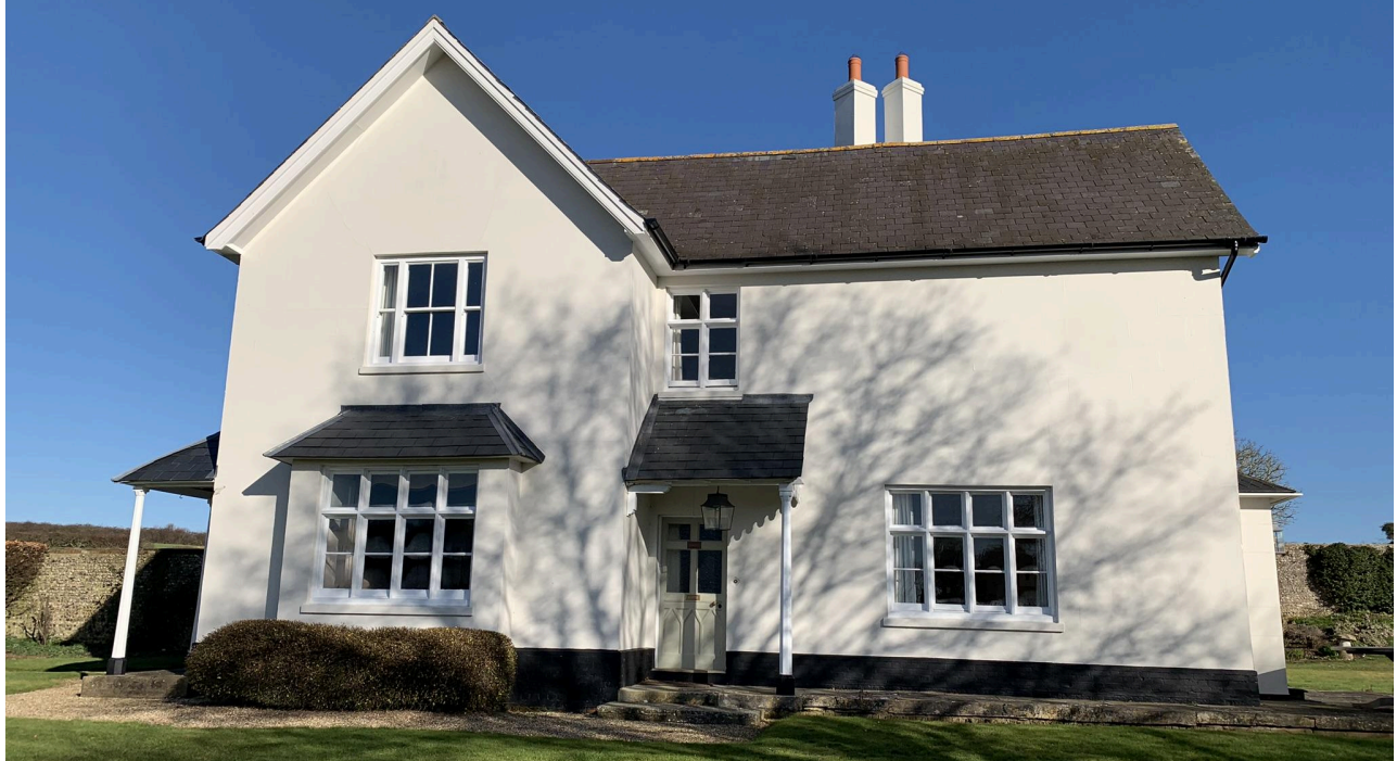
Fig. 3. Original front door to the southern half of the house.
