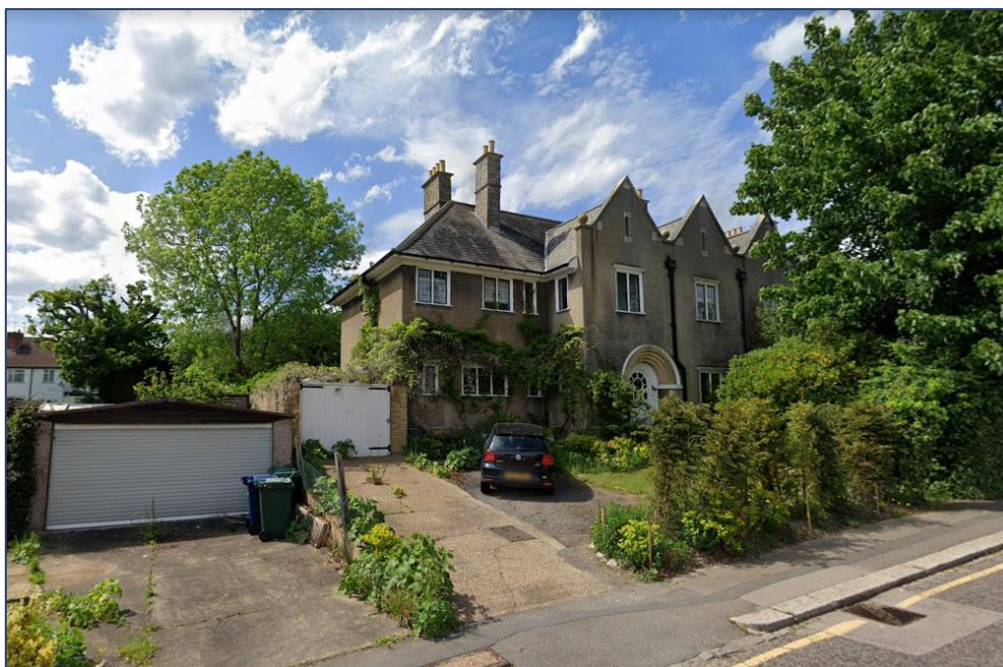
Figure 4- Street view image of 26 Manor Road looking north
