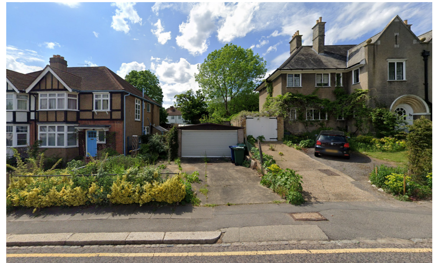
Street view showing the existing garage at No.25b. Looking East.
