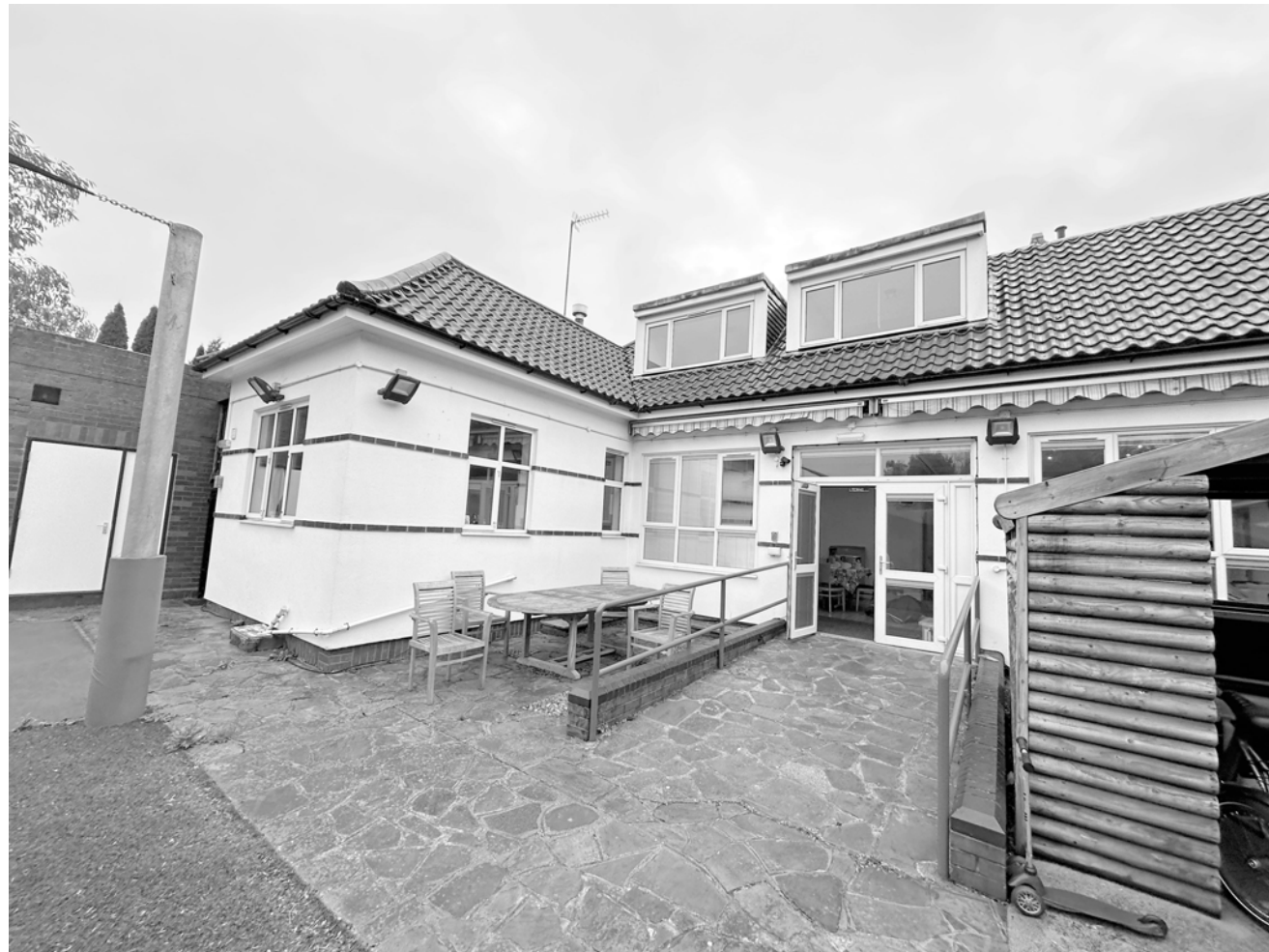
View of rear
