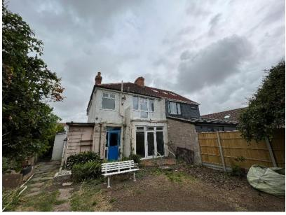
B1 – southwestern elevation There are approximately 10-20 raised tiles located on the south-western roof alongside two missing tiles. This could allow access for crevice dwelling bats to roost between the tiles and the timber roof lining. It could also allow void dwelling bats access into the loft space. The mortar along the ridge tiles appears to be in excellent condition with no gaps.
