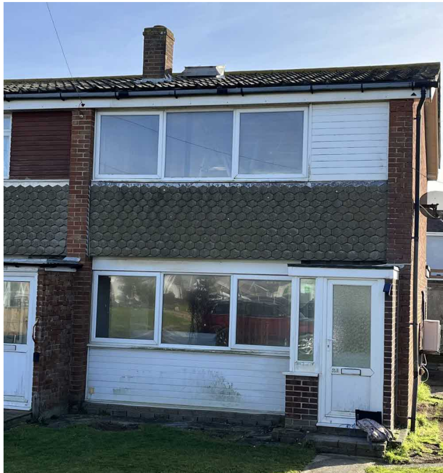
Figure 2. Western elevations looking east.
