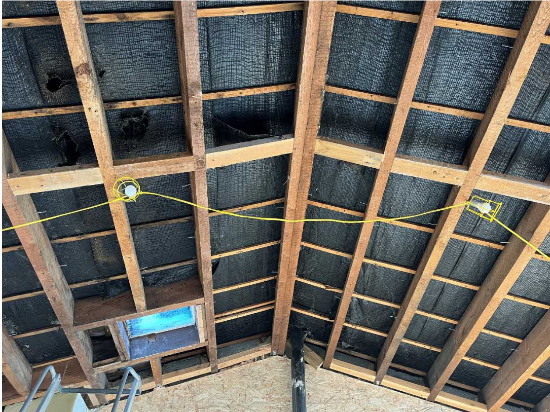
Figure 3. Roof interior view from upstairs living space, looking west
