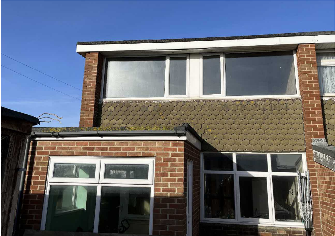
Figure 1. Eastern elevations of 23 Downview Close looking west.
