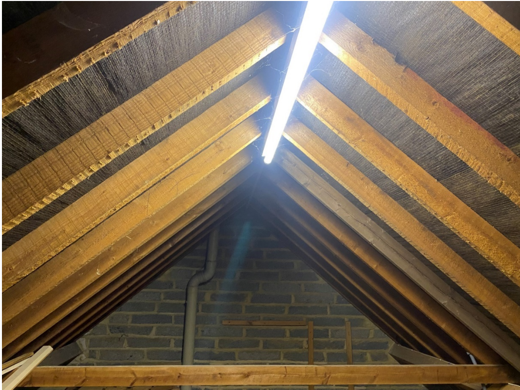
Figure 3. Interior of main roof with modern linings and timber framework.
