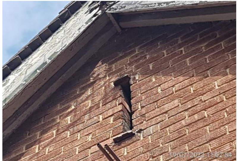
B1 – southeastern gable vent (pictured opposite).
