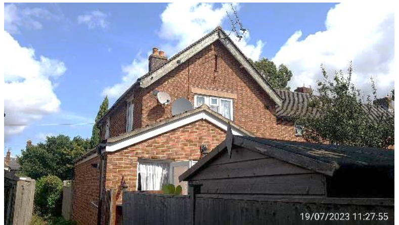
B1 – southwestern and southeastern elevations (pictured opposite).
