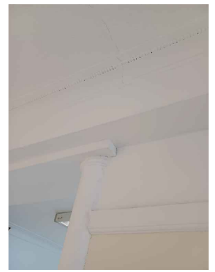
EXISTING PICTURE RAIL
