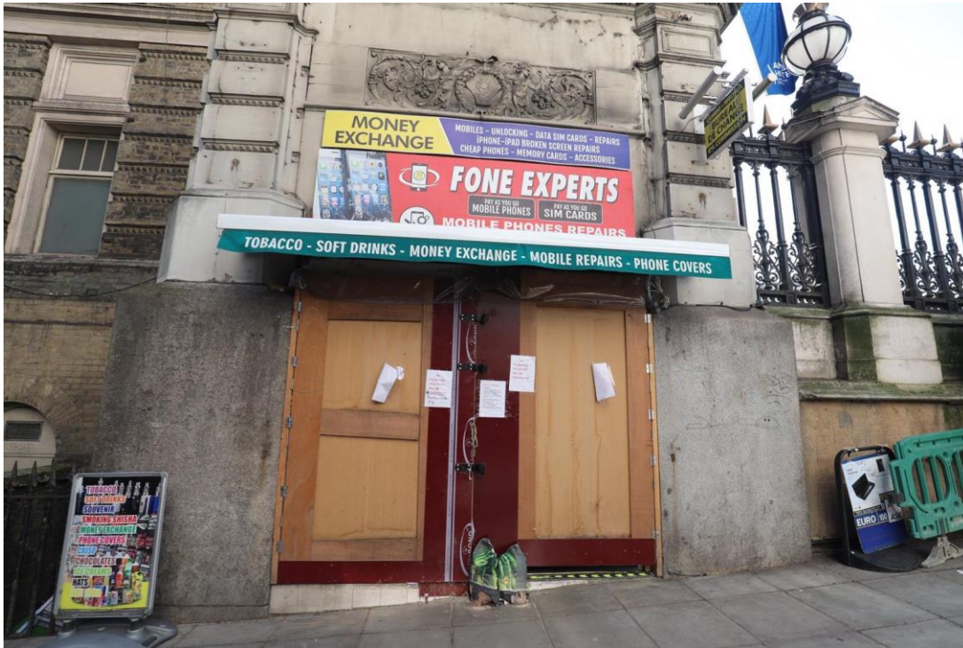
Fig. 8 – Current shutter doors with unfinished/unpainted sections and dilapidated appearance.
