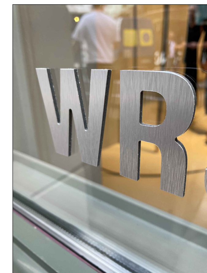
Logo: Milled letters made of 5mm aluminum dibond
