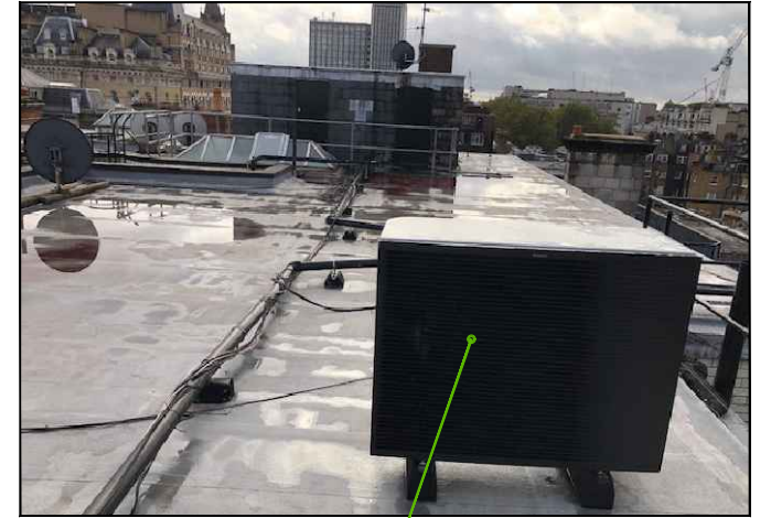
EXISTING AIR SOURCE HEAT PUMP UNIT (OTHER FLATS)
