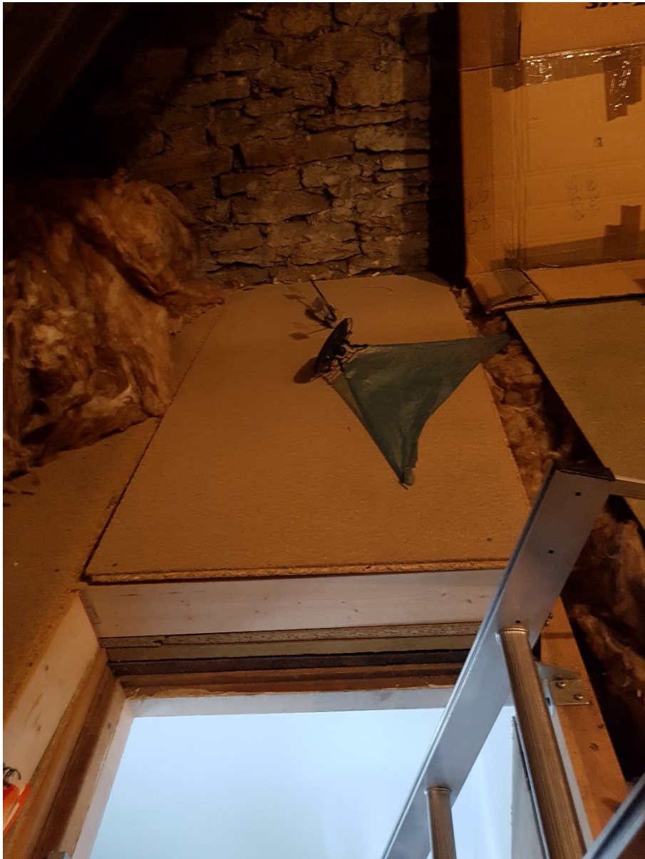
Attic – modern timber floor structure and boarding.
