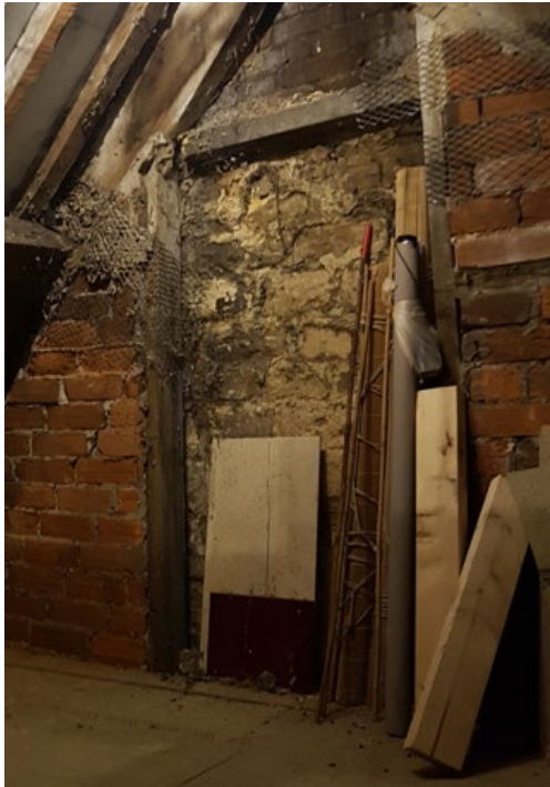
Blocked doorway in loft.
