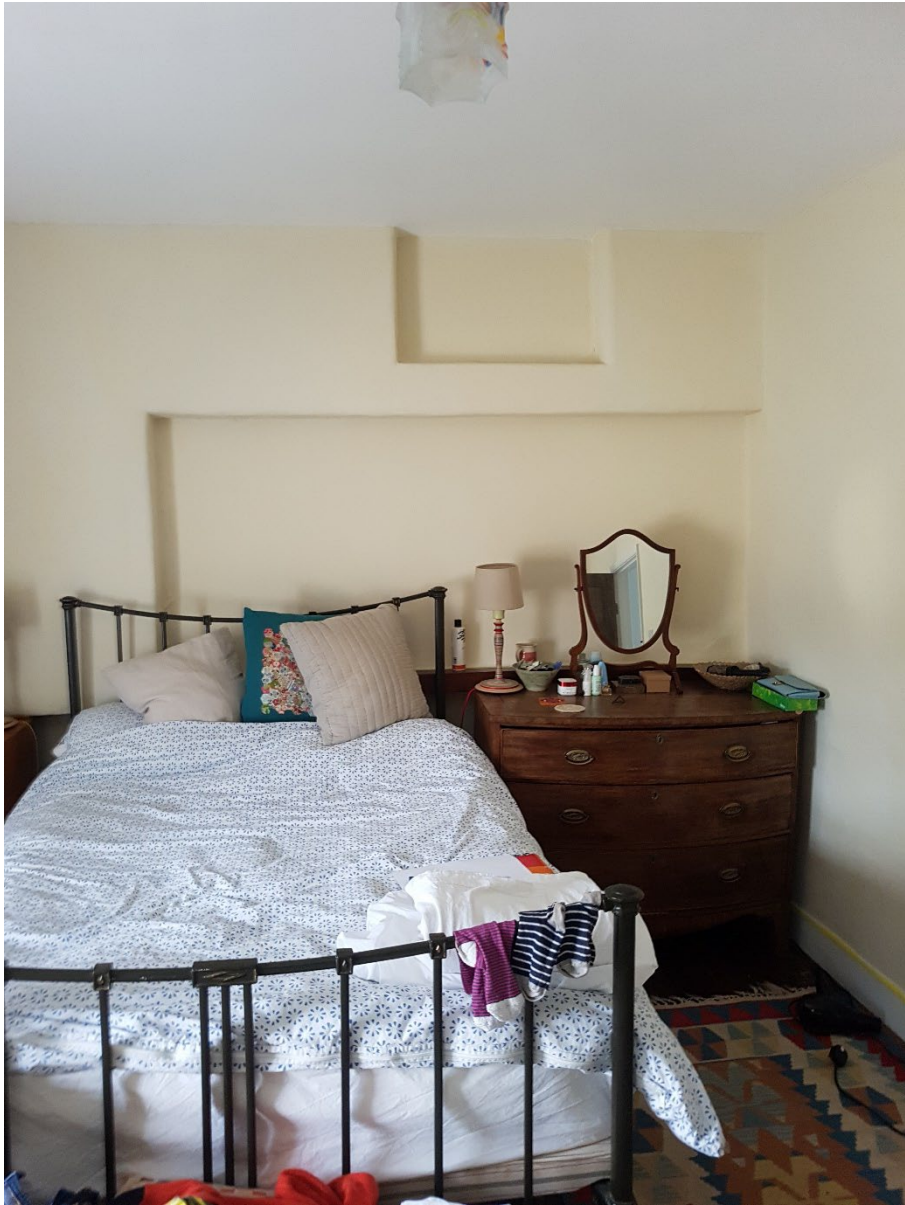
Master Bedroom showing the former opening in the gable wall.
