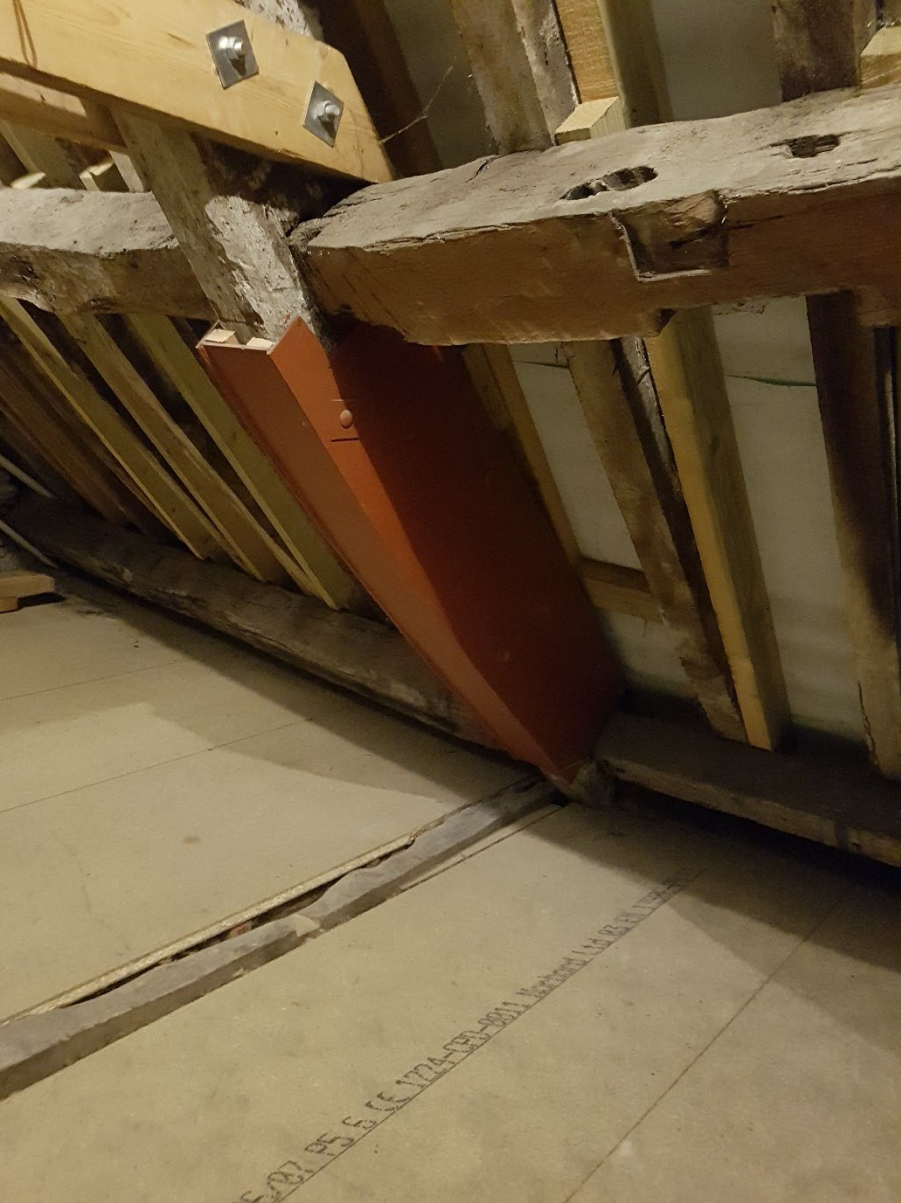
Attic – previous structural works necessary to retain the roof truss.
