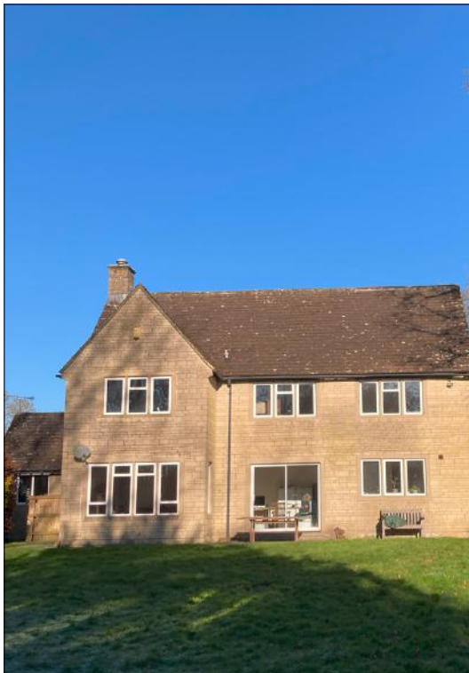
South Elevation Photograph
