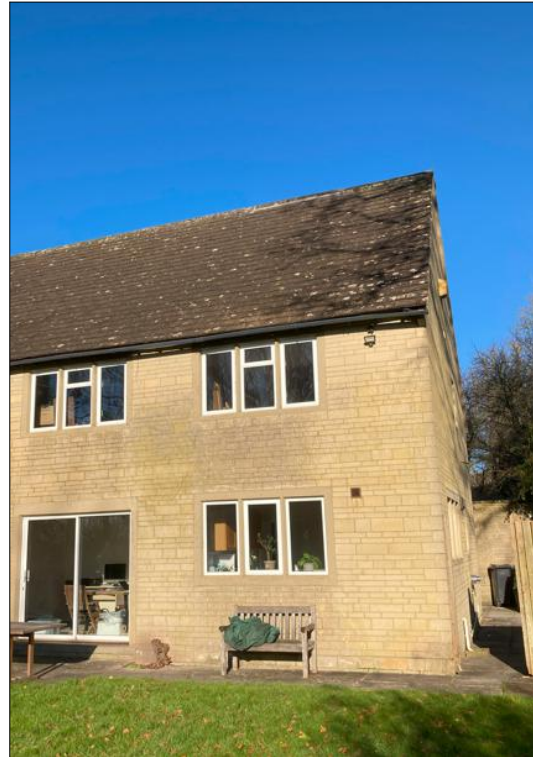
South Elevation Photograph
