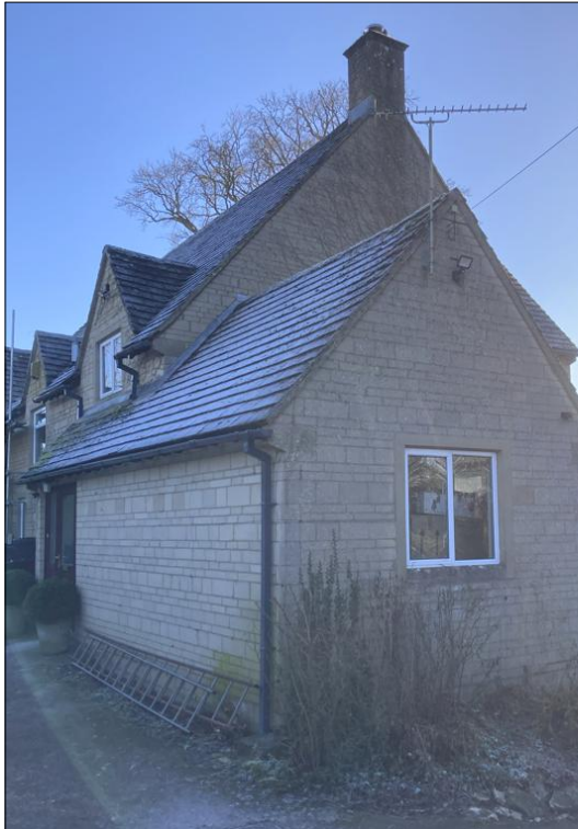
West Elevation Photograph
