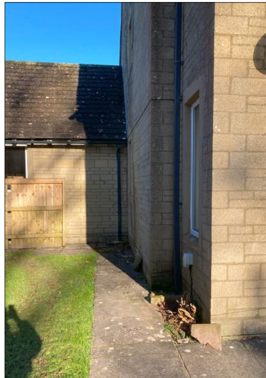
South Elevation Photograph
