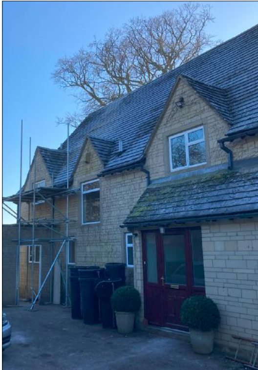
North Elevation Photograph
