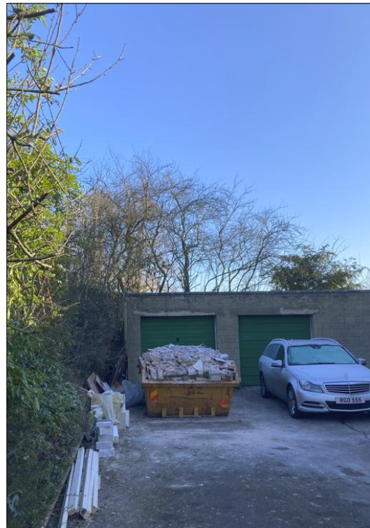
Garage West Elevation Photograph
