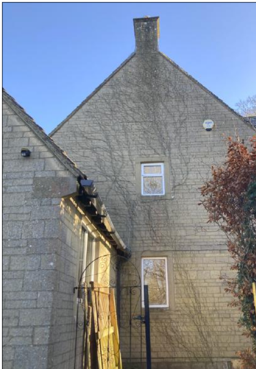
West Elevation Photograph
