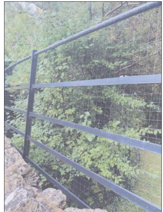
Fig.4 – Precedent Photograph: the image shows the proposed metal agricultural railings to sit behind the boundary wall.
