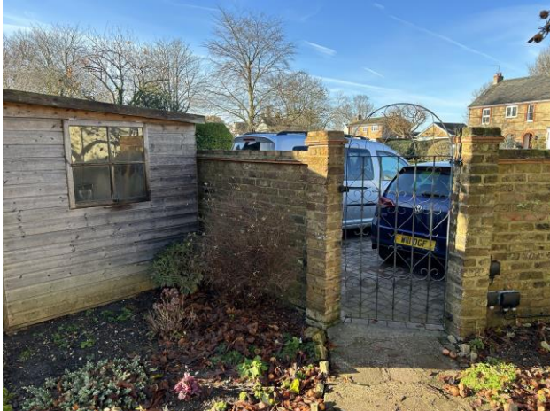
Photograph of the existing garden shed to be removed
