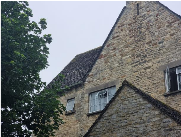
Photograph 3. The northern elevation of the building.
