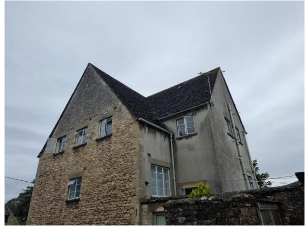
Photograph 2. The building viewed from the south-east.
