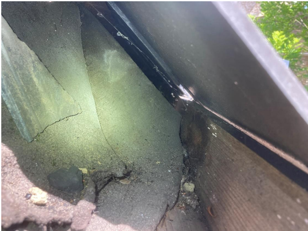
Photograph 4- Open cavity under damaged section of slates
