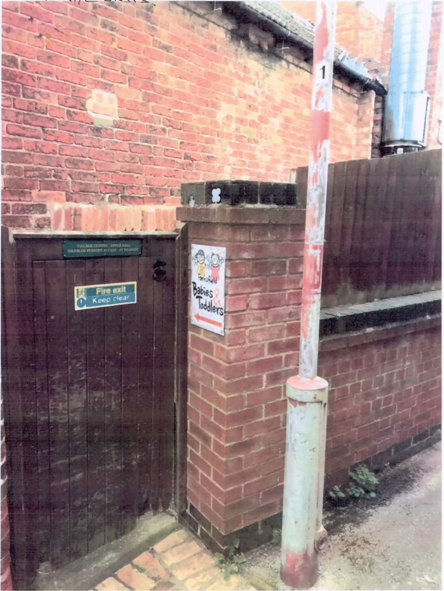
ATTACHMENT 1.4.2 PHOTO SHOWING REAR CONTROLLED ACCESS TO A/C UNITS.
