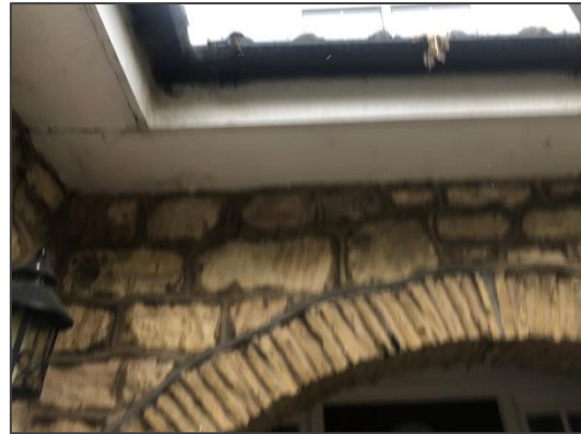
Photo 4: example of well-sealed soffits.
