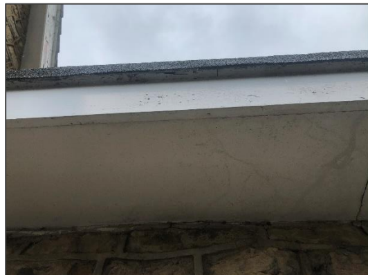
Photo 6: well-sealed flat roof of Building 2.
