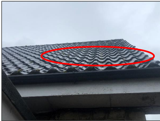
Photo 5: Very low number of slightly lifted tiles.
