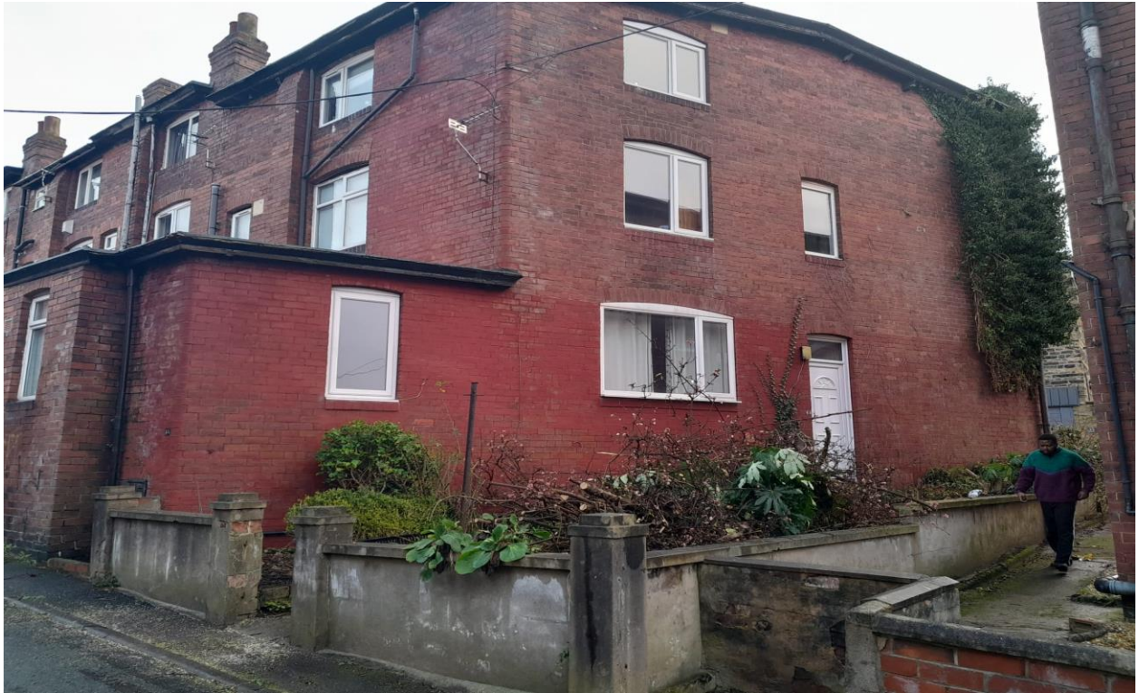
Side entrance and garden area for No.44a.
