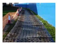
Ground Protection GP2 - Option 1 Where pedestrian-operated plant up to a gross weight of 2t are forecasted, proprietary, interlinked ground protection boards are available, such as DuraDeck or Ground Guard. These can limit compaction when installed with compressible subsurface.
