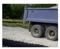
No Dig-Ground Protection GP1 - Option 2 For high use areas or were heavy vehicles are expected, substitute traditional dig out and compacted stone infill with an above ground Cellweb or similar, to avoid the need for excavation and limit compaction – may be retained as a porous sub base for hard Surfacing within the scheme.
