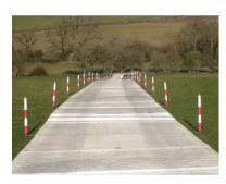
No Dig-Ground Protection GP1 - Option 1 For lower traffic areas, where heavy vehicles are expected, substitute compacted stone infill with a temporary above ground Trackway. This avoids the need for excavation and limits the weight of material build up and limits compaction when installed with compressible sub-surface.
