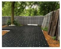
No Dig-Ground Protection GP1 - Option 3 Void forming system such as Permavoid or ArborRaft act as a protection to the tree roots and avoid the need for excavation. These systems also limit the weight of material build up and can be installed with compressible subsurface. – may be retained as a porous subbase for hard surfacing within the scheme.
