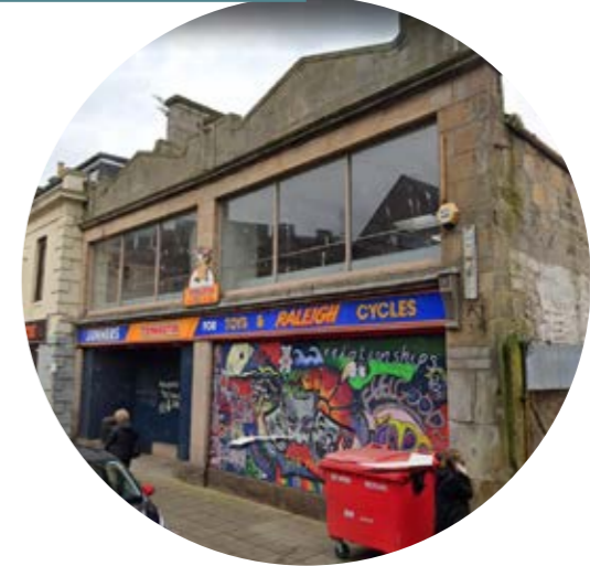
No. 51 Art Deco Facade
