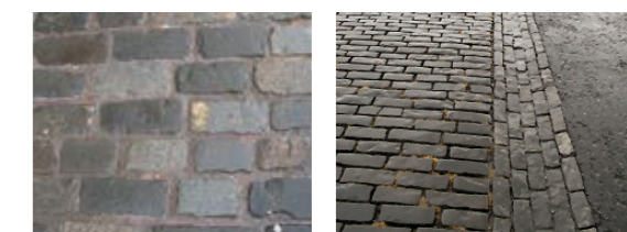
Vehicle Area - Asphalt Surfacing with Whin Sett Detail
