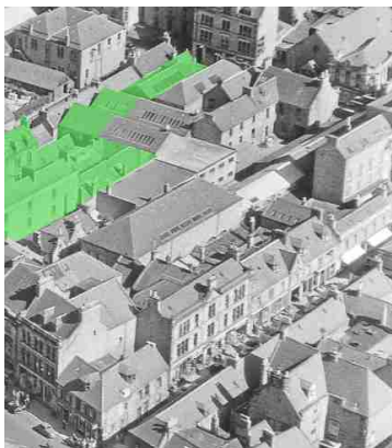
Demolition of properties at the rear of 51 South St, to facilitate the redevelopment of the Gordon Arms Hotel in 1966, are highlighted in Green.
