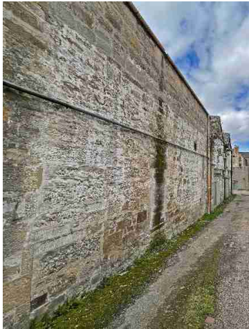
SS.02-04a: 51 South Street – Return Wall
