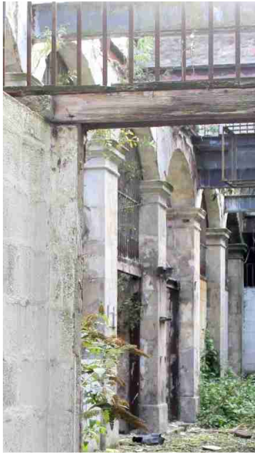
SS.02-05a: The ruins of the market arcade, left exposed after a fire destroyed the building.
