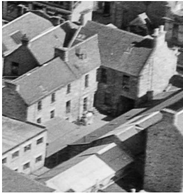
SS.01-02a:- Wing and courtyard to the rear of 53 South Steet in the 1950s showing side entrance.
