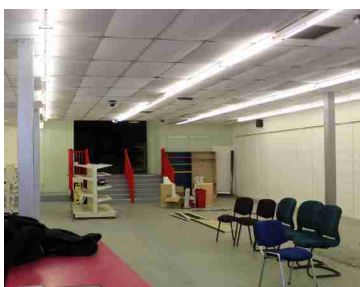
SS.02-01c: OS Map, 25 Inch, 1856 Present day premises at 57 South Street showing modern structural steelwork.
