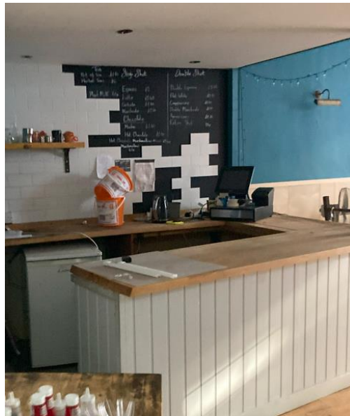
Image 2; Existing bar in the front to be removed and replaced in like for like position with timber top and metal front. Back fitting to be renewed with metal upper back fitting, with new tiles/mirror to wall behind. Metal framed overbar to be fitted above bar front.
