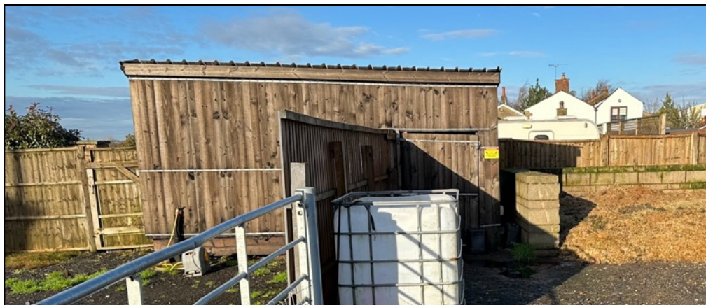
Figure 10 Building B1, a small wooden storage shed near the site entrance
