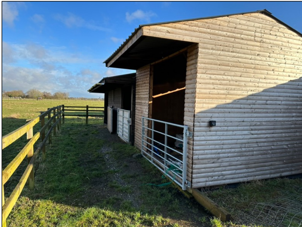
Figure 14 Buildings B8 and B9
