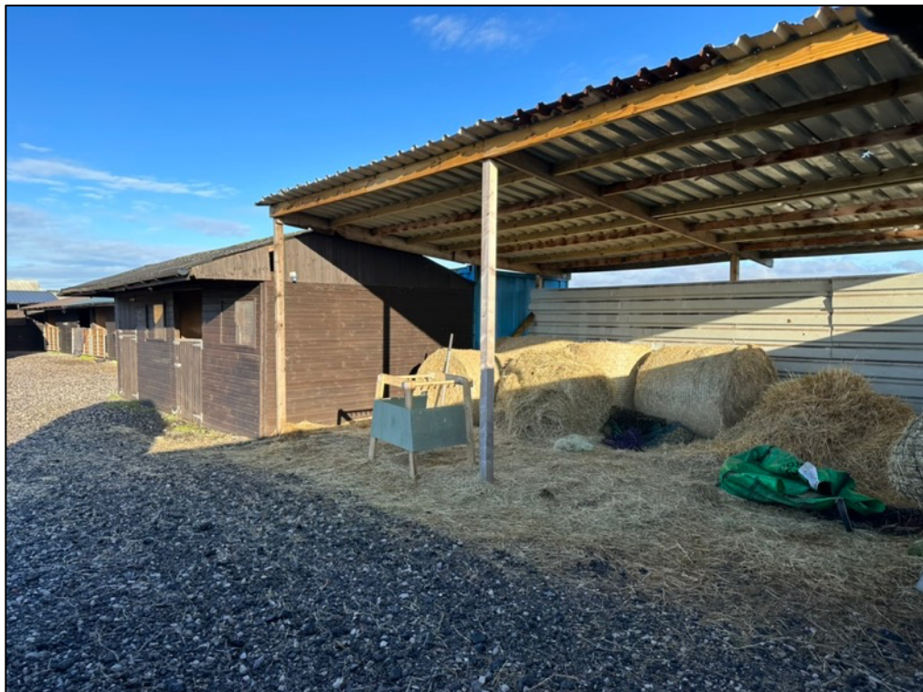
Figure 15 Buildings B13 and B14
