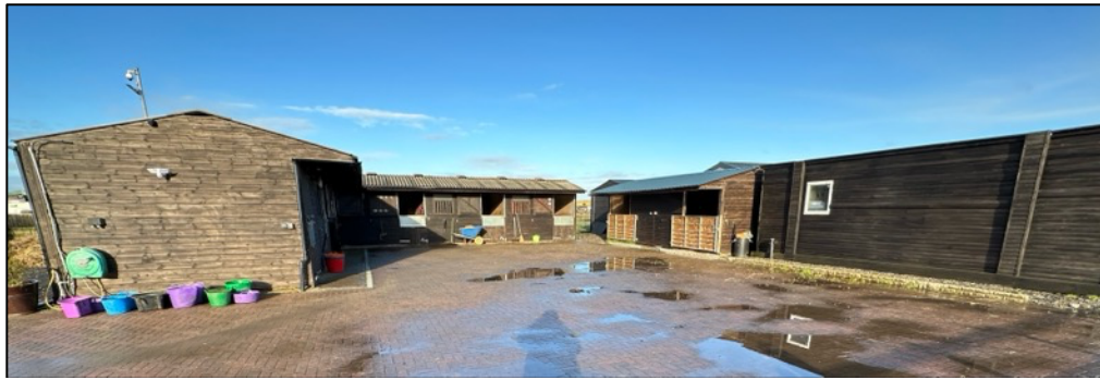
Figure 11 Buildings B2, B3 and B4 as viewed from the east
