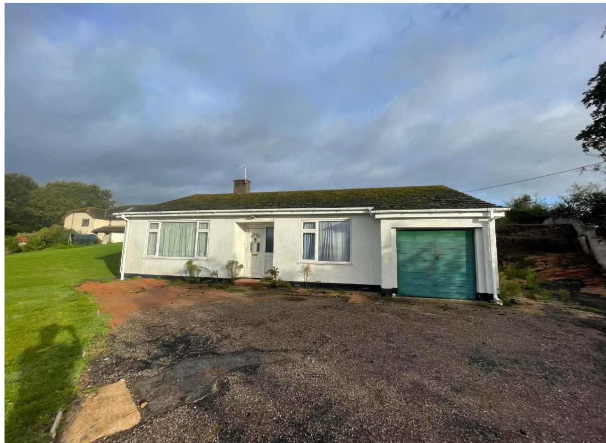
Photograph 1. Timbervale – south elevation
