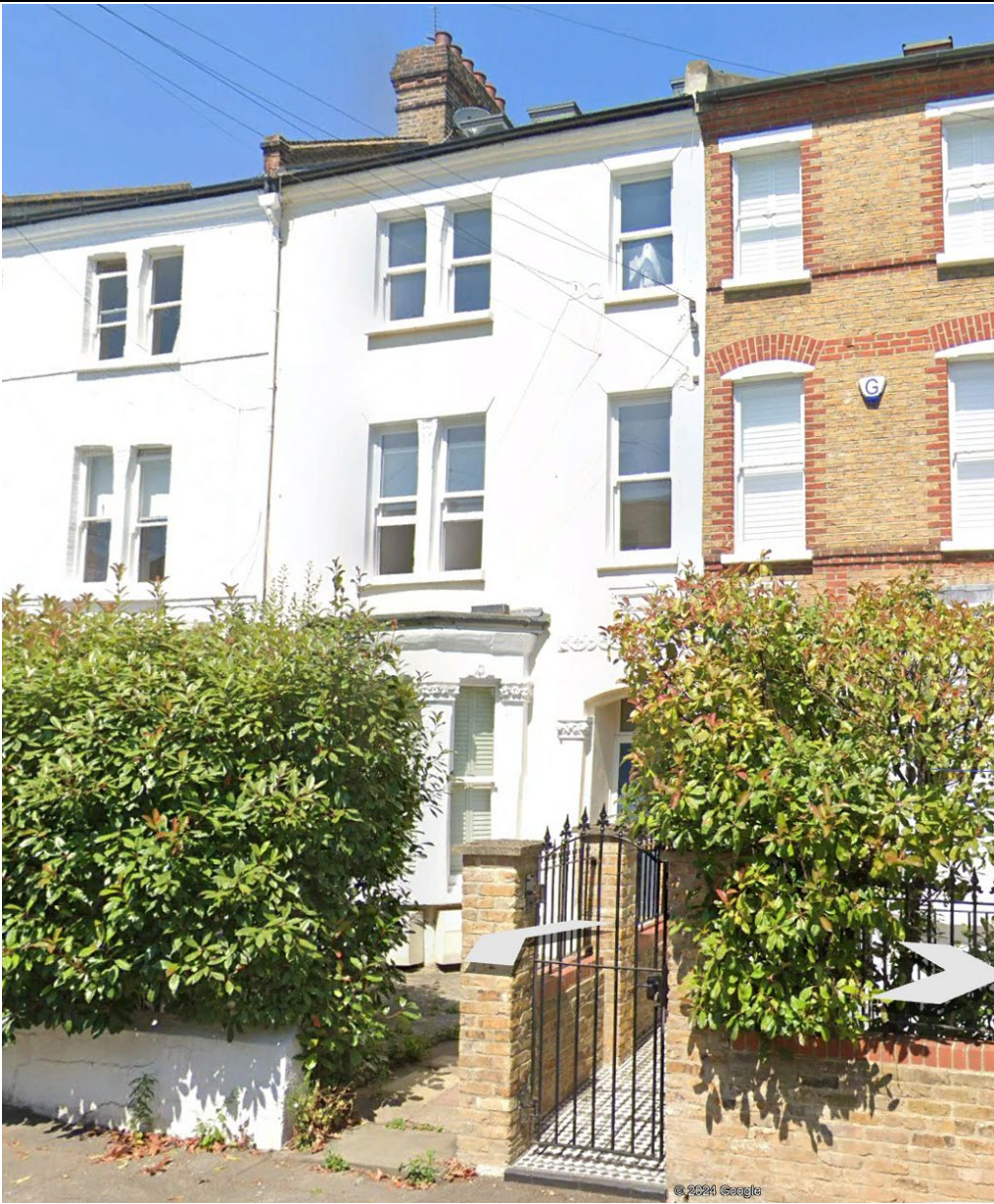
Plate 6 Property frontage looking N
