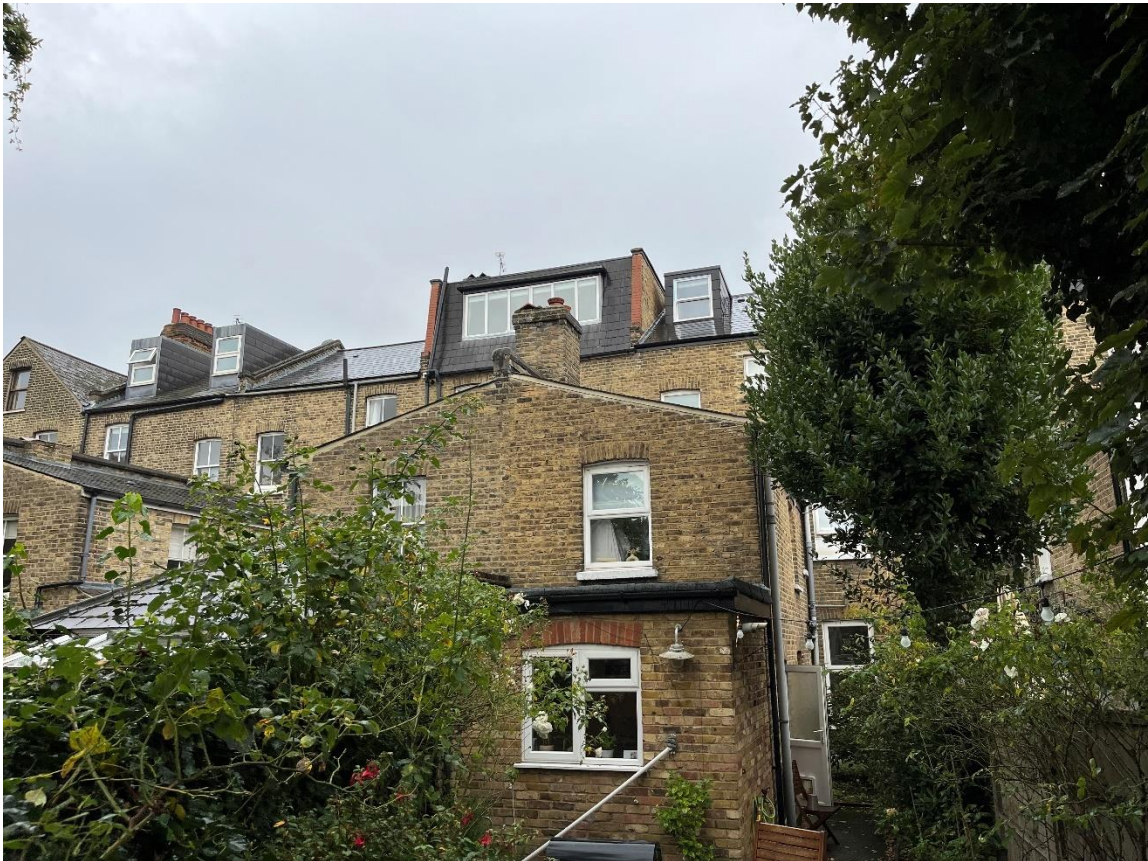
Figure 3,4 – 20 Lydon Road viewed from the rear. Existing rear extension.
