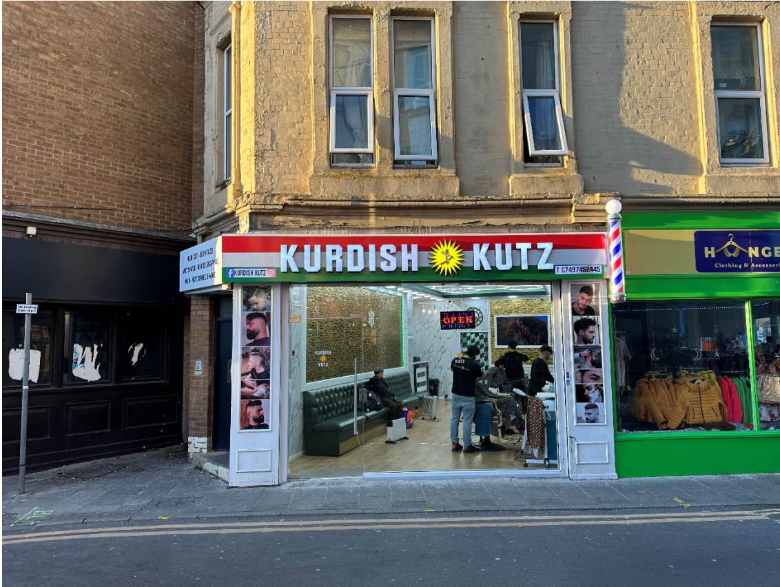
Figure 1. Image of principal elevation
