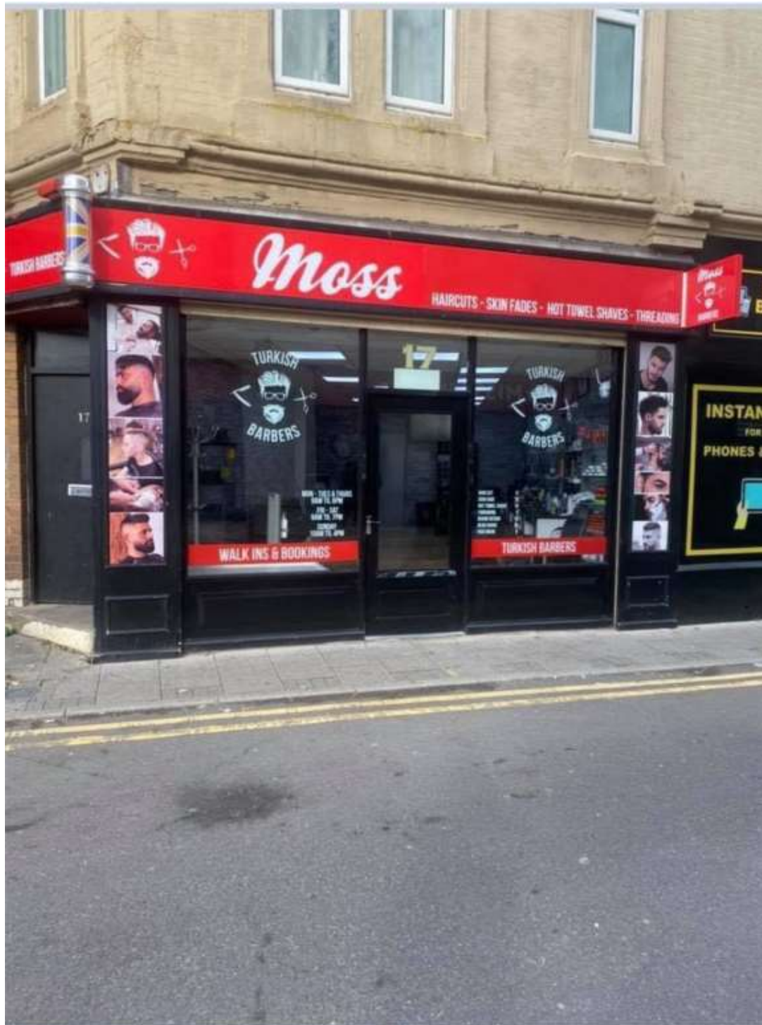
Photograph of previous frontage
