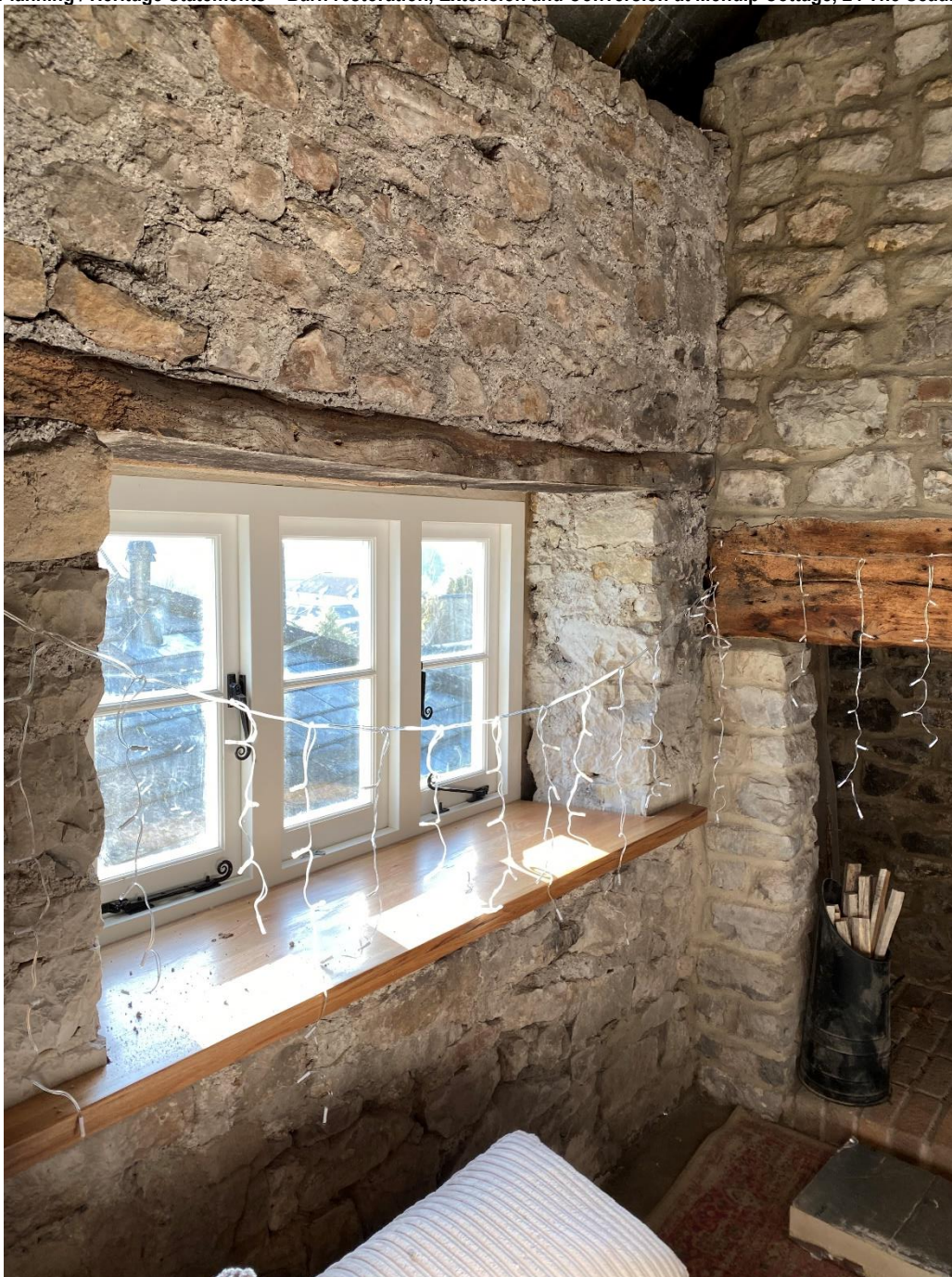
[Previously restored timber framed window unit to main barn area]
