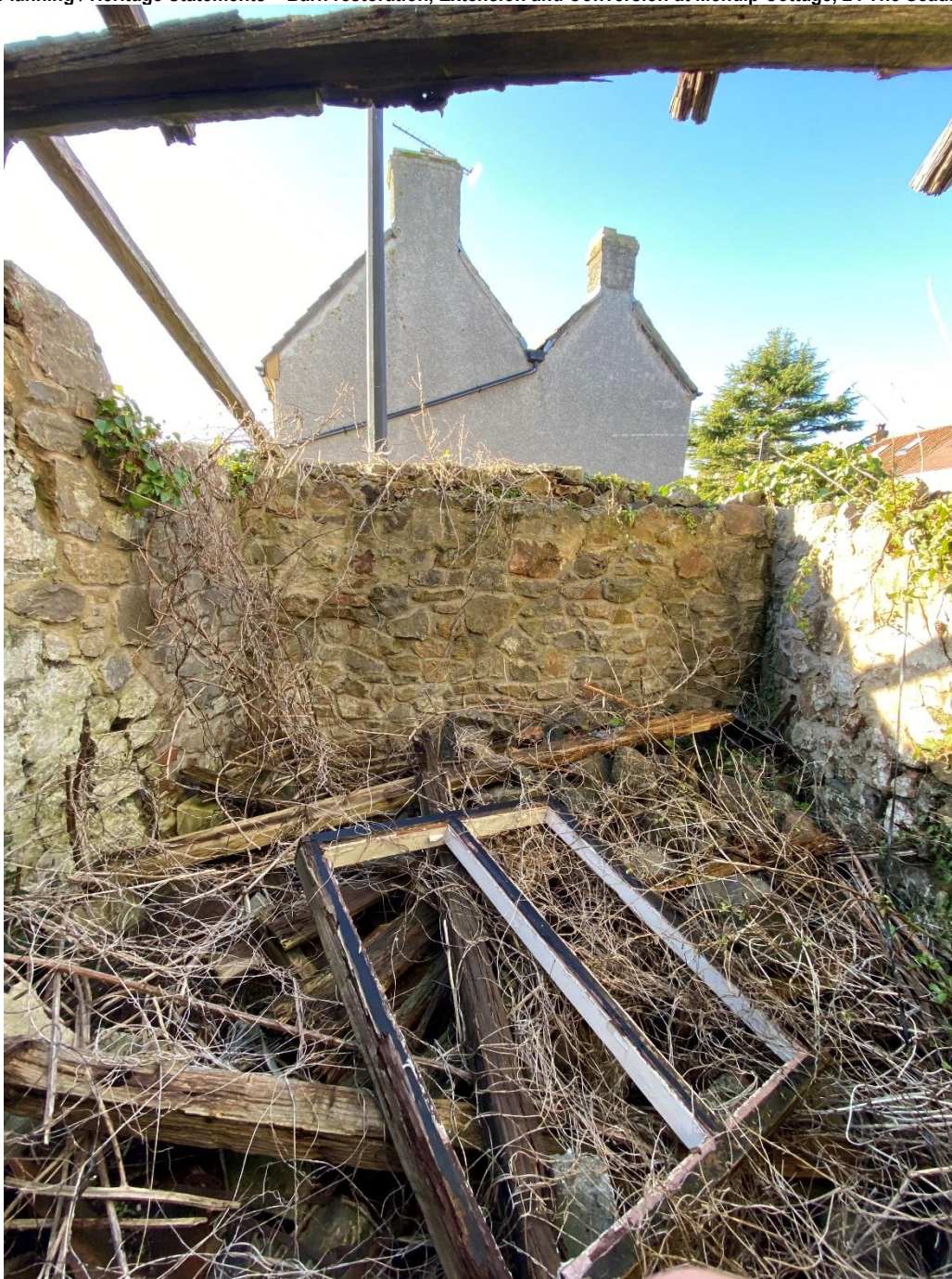
[inside part of the dilapidated adjoining outbuilding – post wall repairs]
