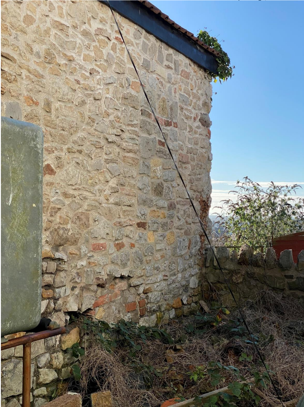
[existing detached barn building and condition of walls as existing]
