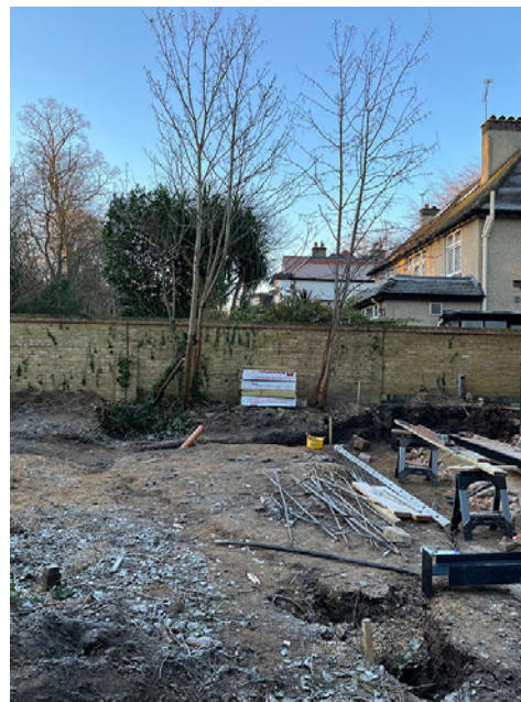
T4 & T5 - proximity to house & wall
