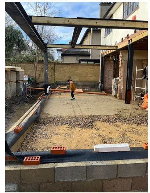
T4 & T5 - proximity to house & wall
