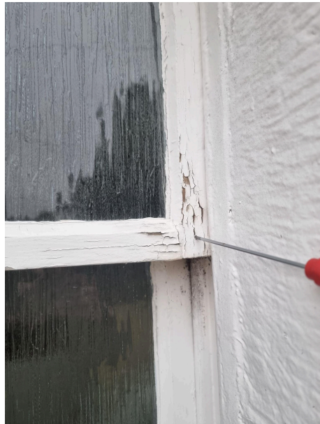
Rotten top and bottom sash
