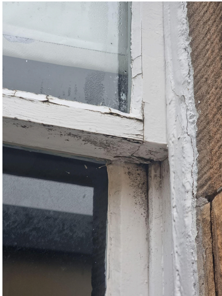
Bokeh tenon joints, putty and mastic.
