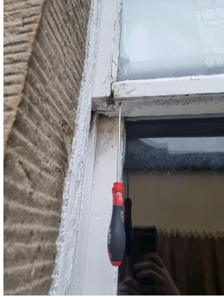
Rotten top and bottom sash
