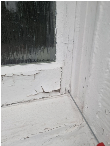
Rotten top and bottom sash
