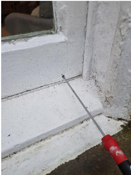
Broken internal putty/paint
