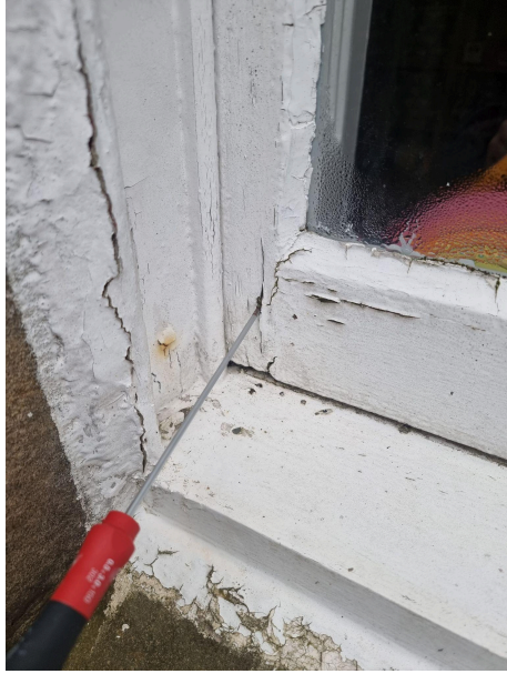
Rotten top and bottom sash
