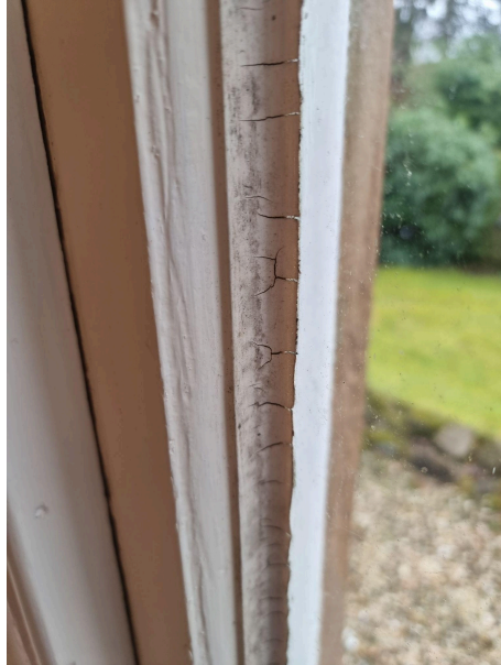
Broken internal putty/paint
