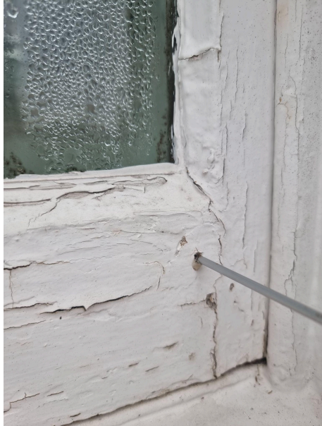
Rotten sash and mid rail
