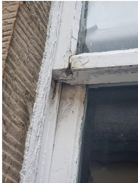
Bokeh tenon joints, putty and mastic.
