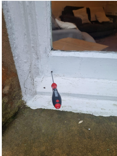
Broken internal putty/paint
