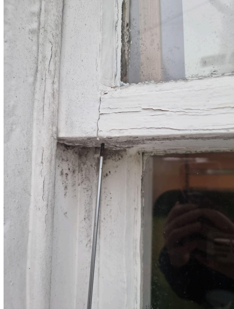
Rotten sash and mid rail
