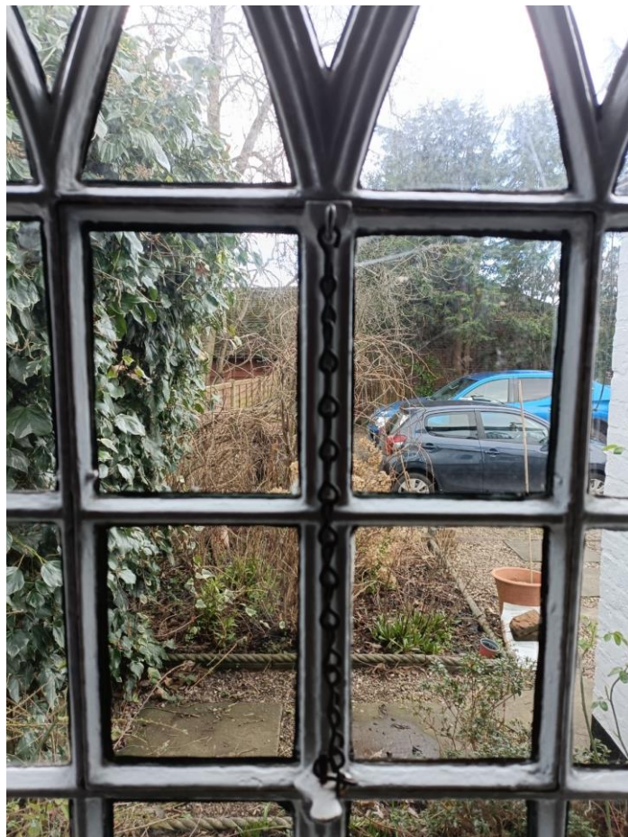
Typical opener detail
