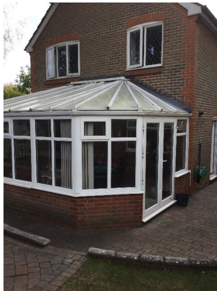
General view of rear conservatory
