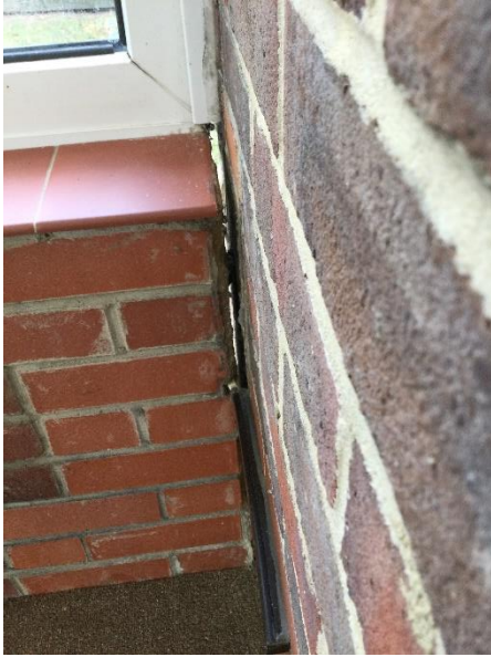
Gap at the junction of the right-hand wall and the main property
