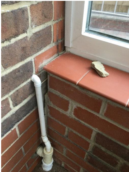
Gap at the junction of the left-hand wall and the main property
