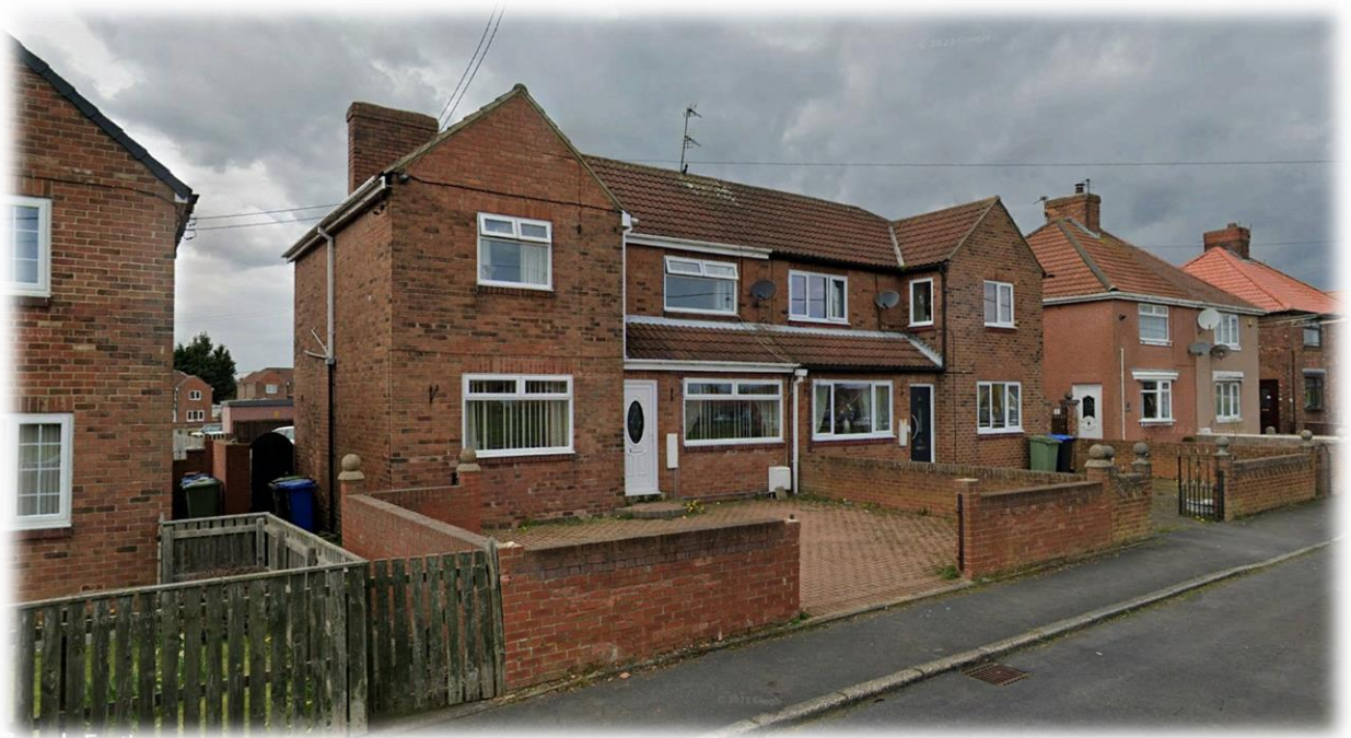
EXISTING SEMI-DETACHED HOUSES OPPOSITE SITE ON JACK LAWSON TERRACE
