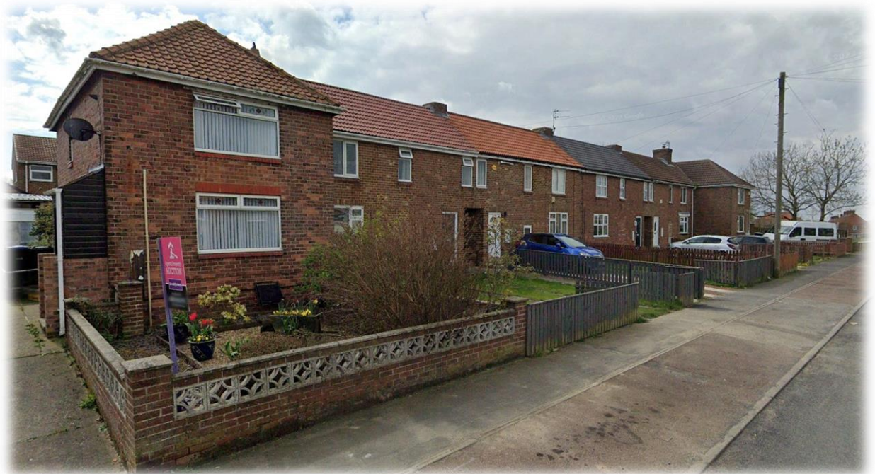
EXISTING TERRACED HOUSES ALONG BYRON STREET
