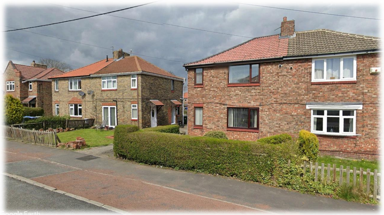
EXISTING SEMI-DETACHED HOUSES ON BYRON STREET
