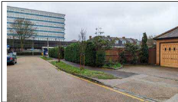
Photograph 1 –The south and east boundaries of the site.
