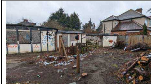
Photograph 5 – Recently cleared small trees that grew through the hardstanding layer.
