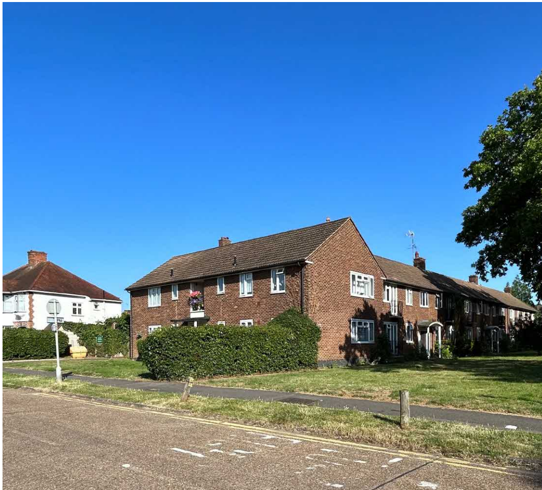
2-storey pitch roof building houses flats with access from Fairmead and Ewell Road.
